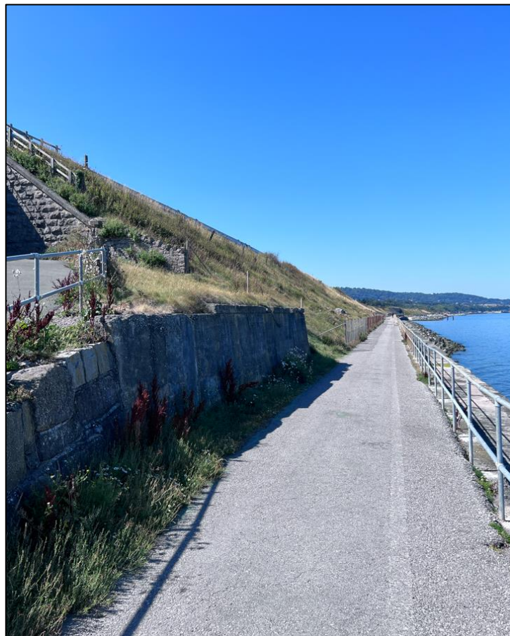
Figure 7: Public footpath situated at the rear of the sea wall, below the rail embankment.
