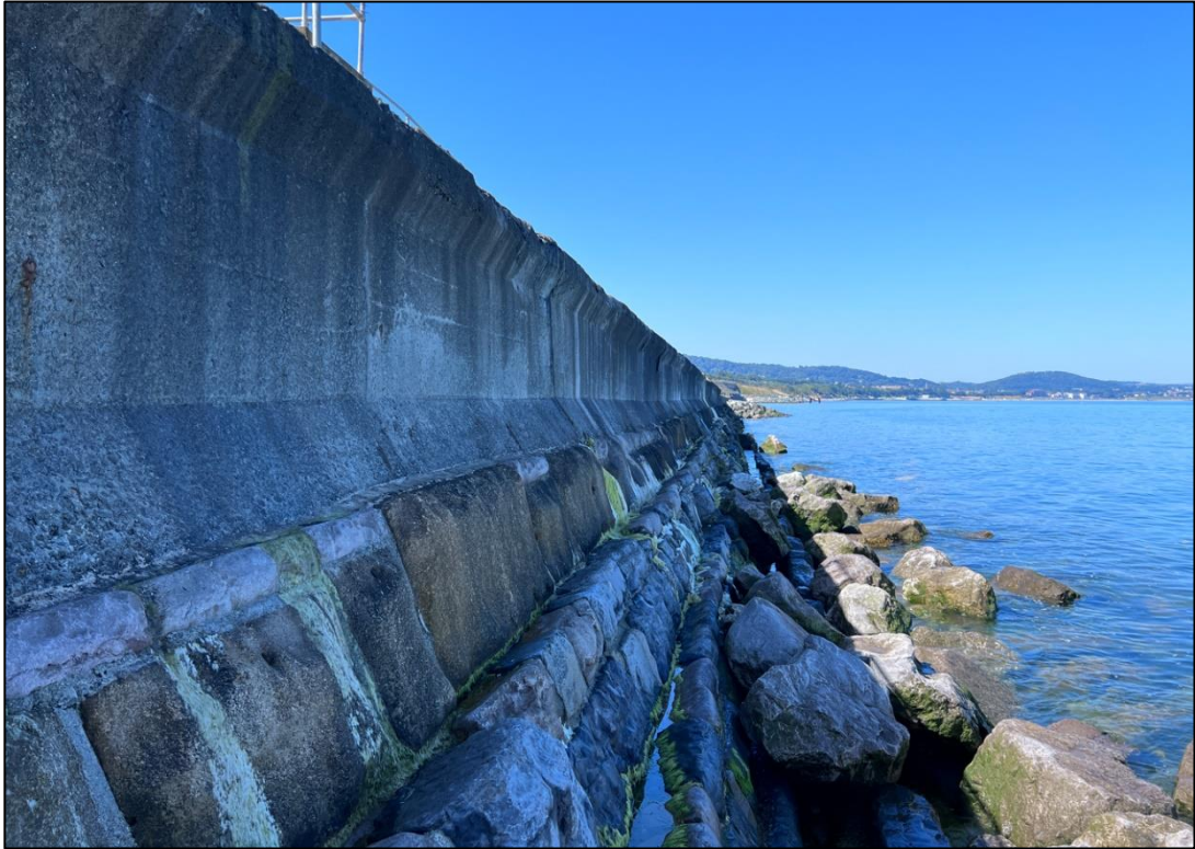
Figure 4: View of tied sea defence facing west.
