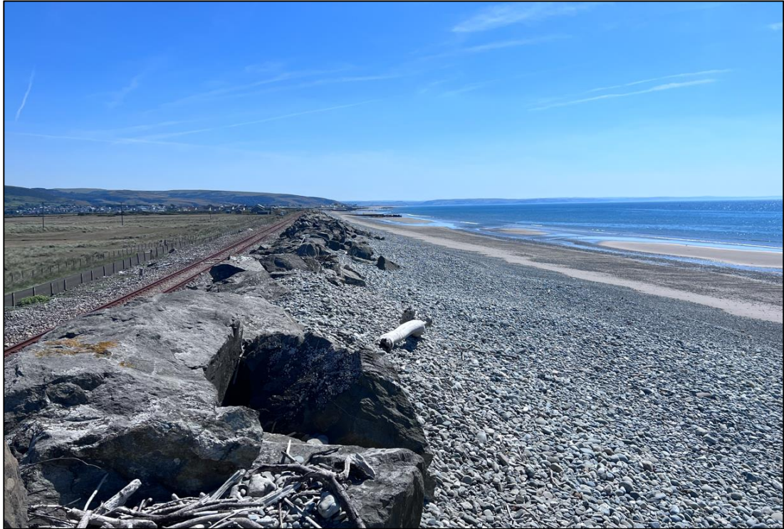
Figure 3: Raised rock armour wall above rail corridor with pebble beach seaward.
