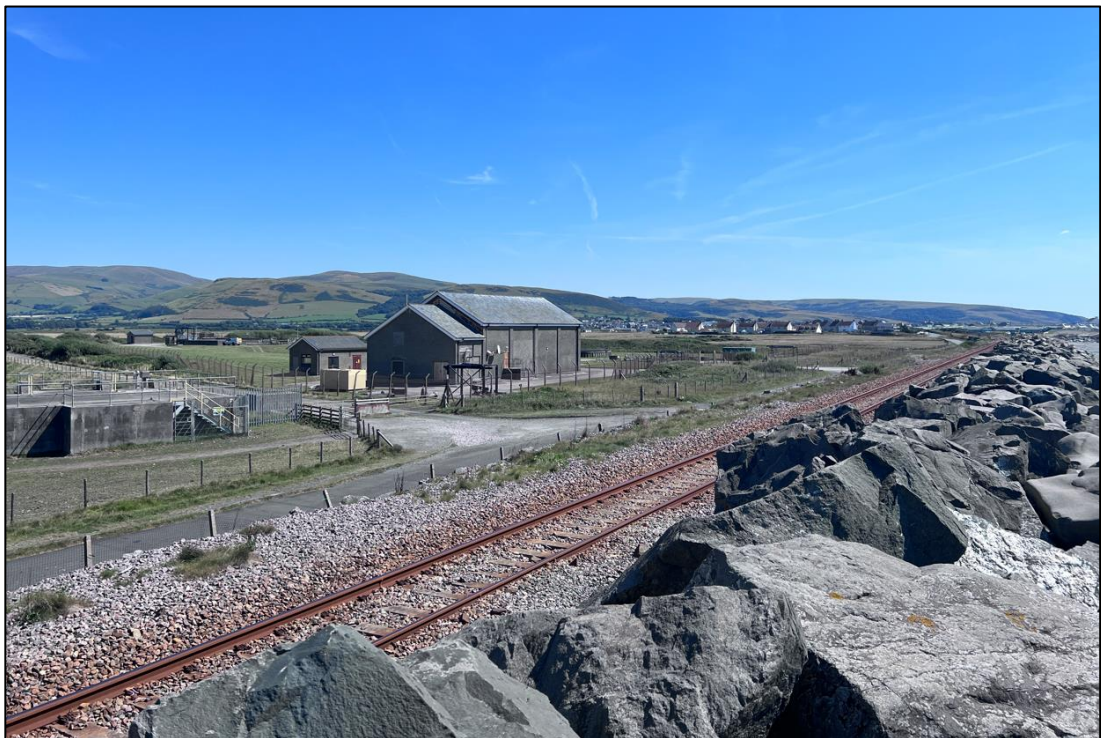
Figure 4: Tywyn sewage works connected to rhyne.
