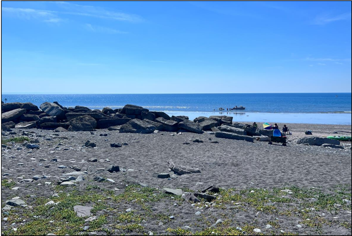
Figure 7: Rock armour separate from main defences further seaward of rail corridor.
