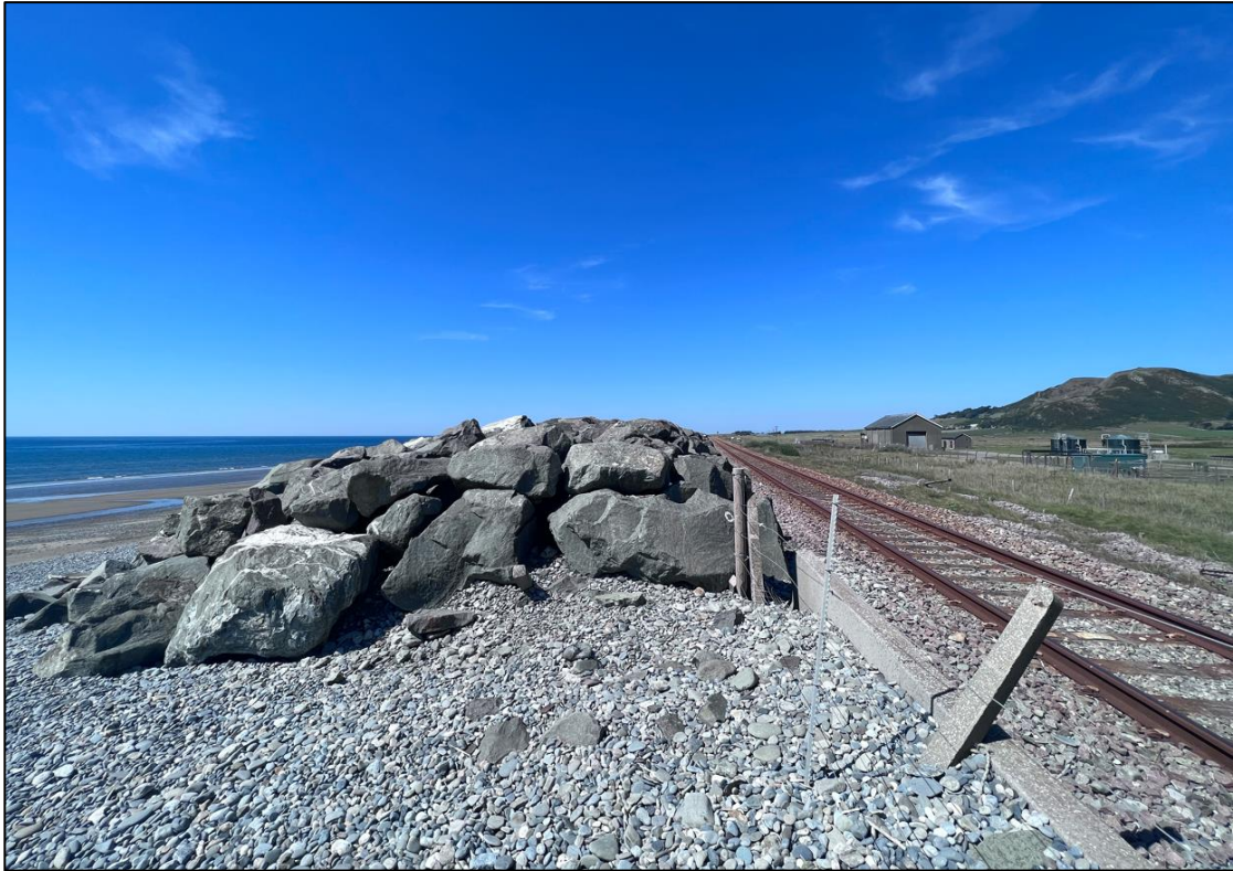
Figure 5: Rock armour along rail boundary ends 100m north of proposed compound area.
