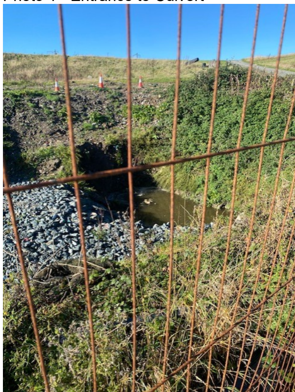
Photo 1 - Entrance to Culvert
