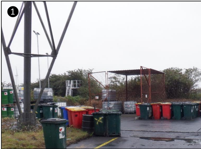
Photograph 1 & 2: IBCs storing waste oil/lubricant not provided with secondary containment.
