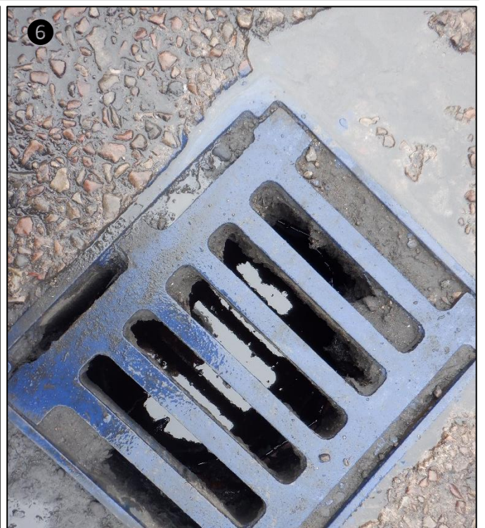
5 & 6: Liquid pollutant contamination of site surfaces and surface water drainage system gully pot.
