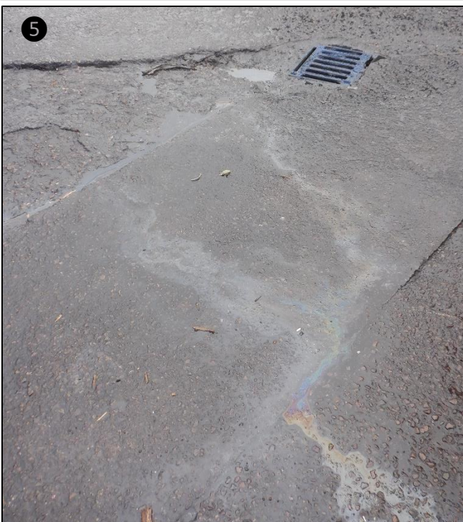
5 & 6: Liquid pollutant contamination of site surfaces and surface water drainage system gully pot.
