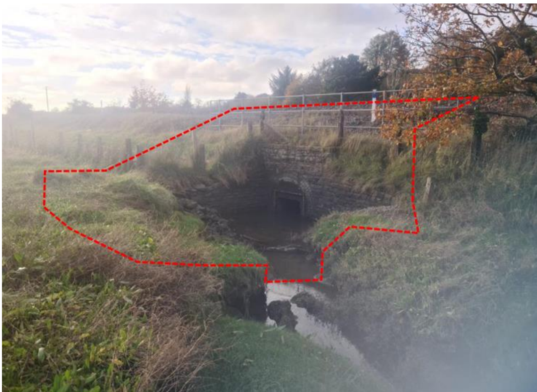
Figure 6: Image of working area highlighted in red.
