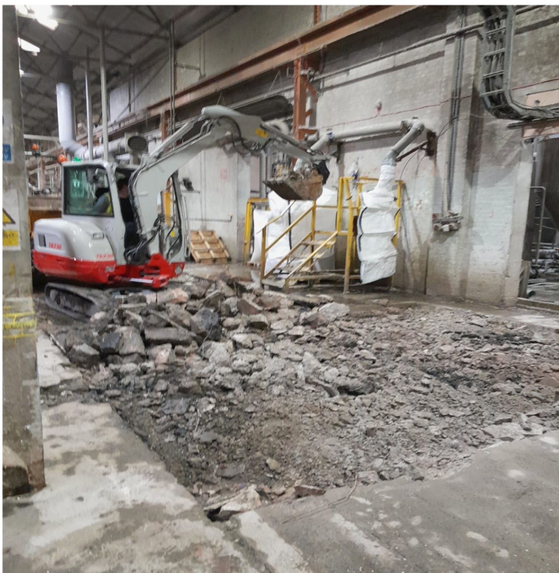
Image 1 - Picture showing the factory floor being resurfaced
