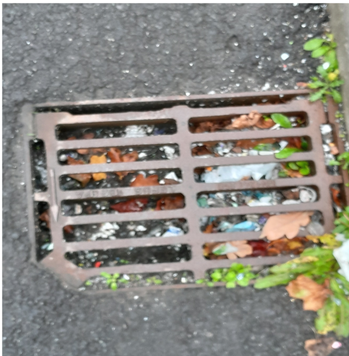
Image 3 - Picture showing congested filter in drain
