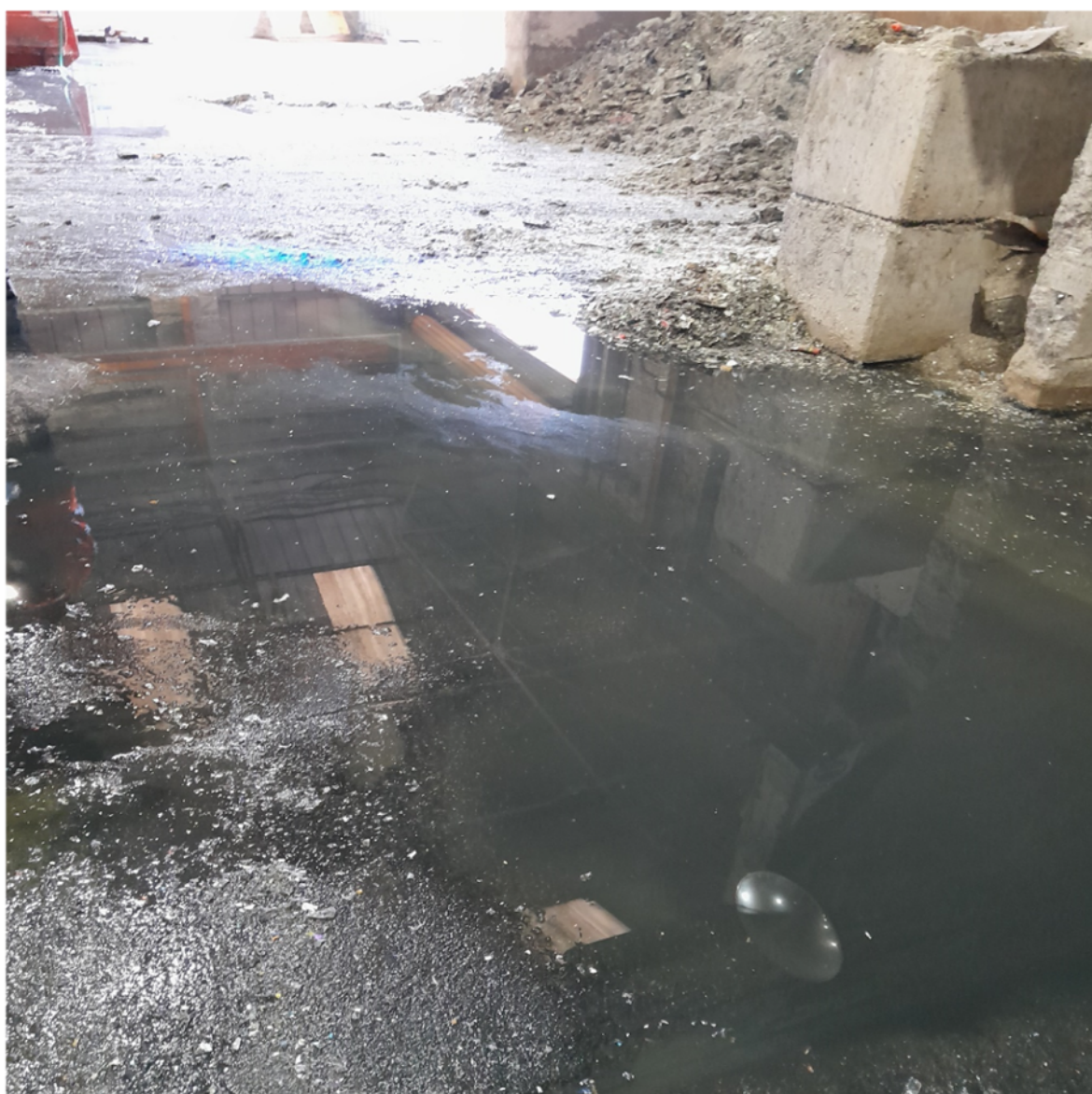
Image 2 - Showing water soaking out of wastepaper sludge pile
