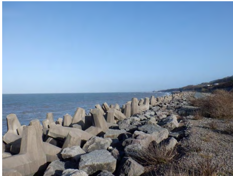
Plate 1 – General view of CMU 3-1 looking north east including revetment and coastal cycle path.
