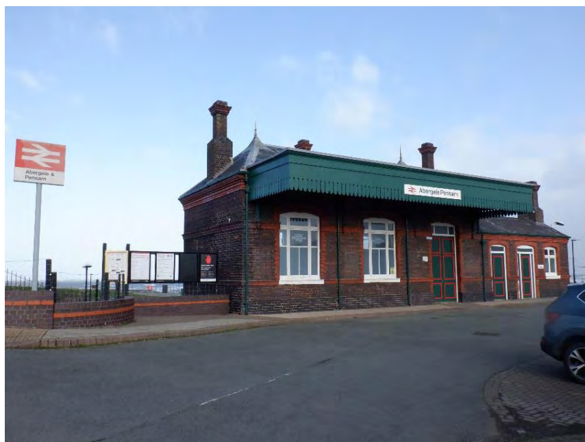
Plate 23 – Abergele and Pensarn Railway Station Booking Hall (18703) facing north west.
