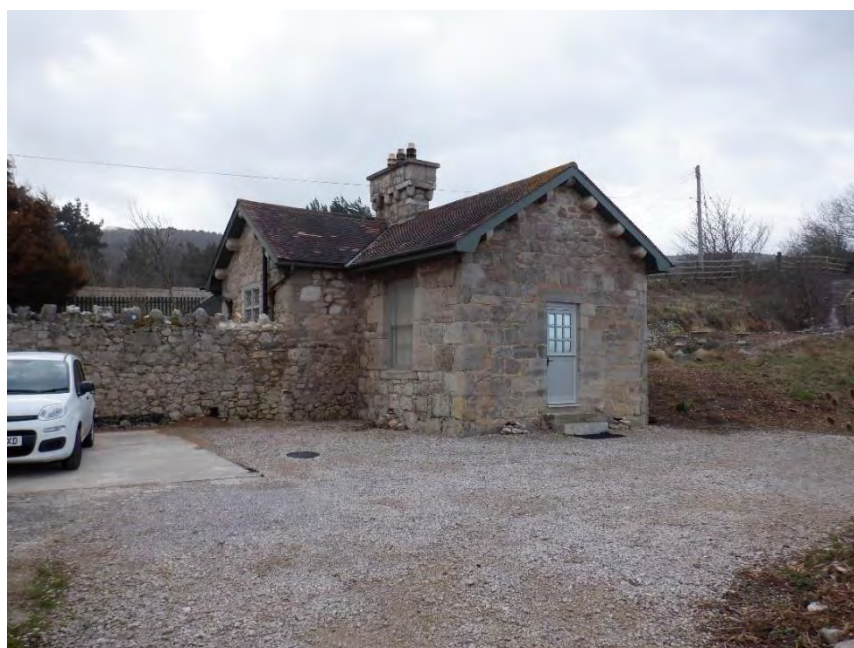
Plate 16 – The new heritage asset identified in CMU 3-3, Ty Crwn (JBA-1), the historic bathing house of the Lloyds of Gwrych, facing south west.
