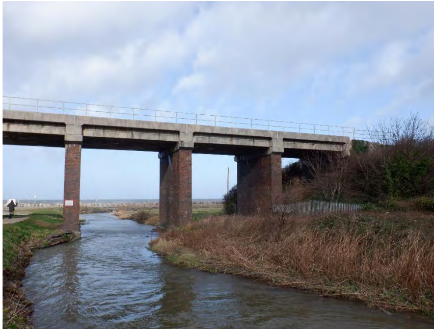
Plate 11 – The Dulas Railway Viaduct (87069) facing north.
