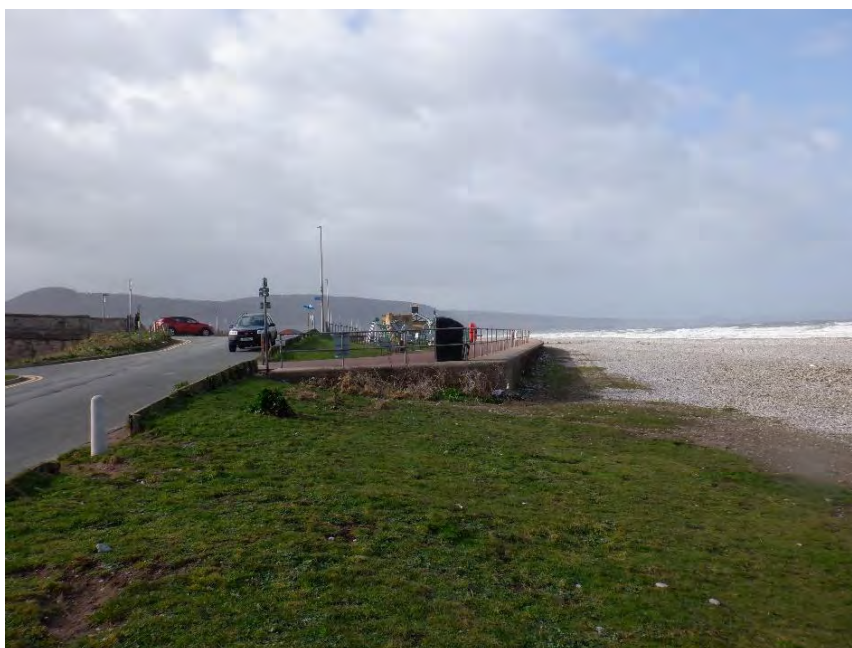
Plate 21 – View from the eastern side of CMU 3-4 facing west.
