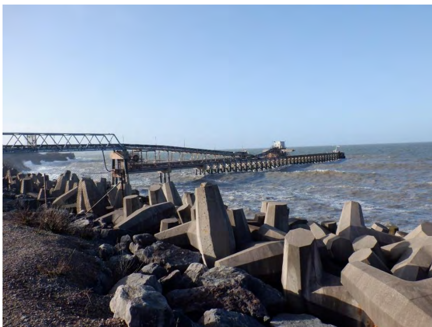
Plate 5 – View of the Raynes Quarry Jetty (34205) from the cycle path facing north west.
