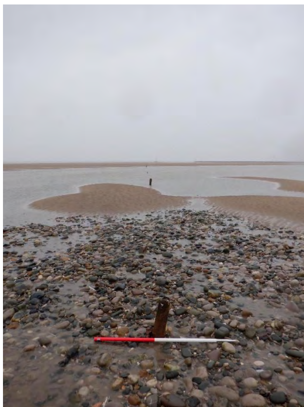
Plate 39 – Remains of a groyne system that were identified in the eastern side of the CMU facing north east at Foryd Harbour
