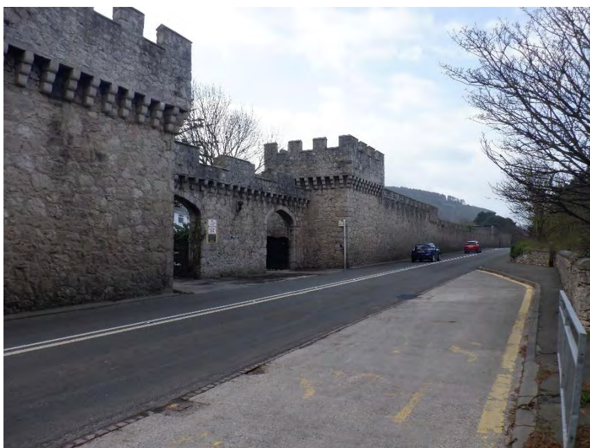
Plate 18 –Hen Wrych Lodge (19039) facing south west.
