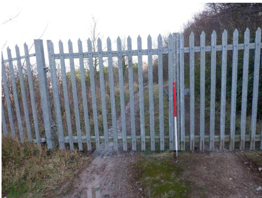
Plate 3 – Locked access to the Llysfaen Post Medieval Railway Station (87072) facing north east.
