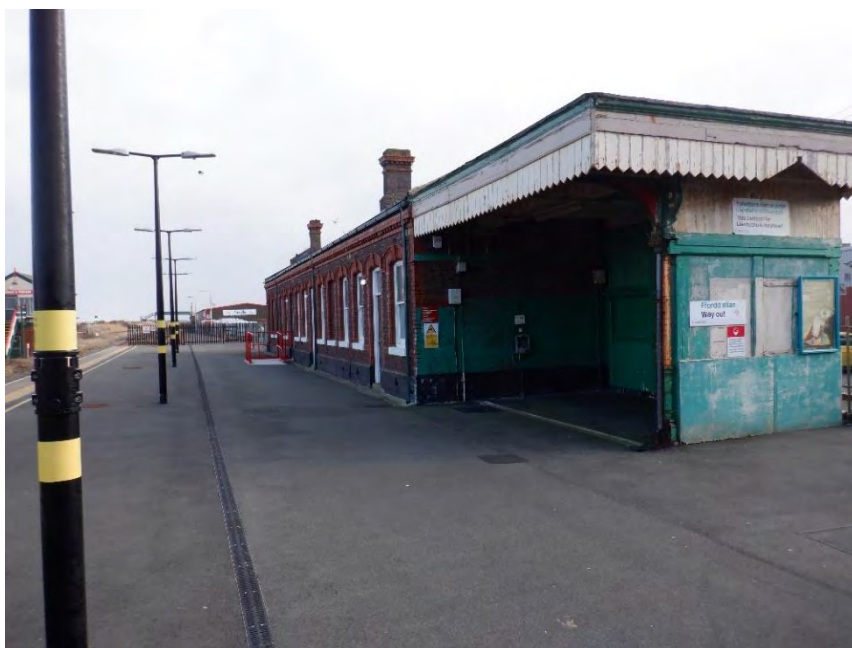
Plate 25 – Abergele and Pensarn Railway Station “Down” Platform building (18705) facing south east.
