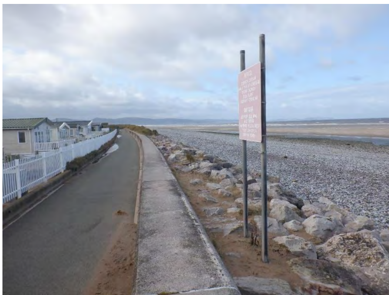
Plate 38 – The view looking west across CMU 3-5C back along Kinnel Beach.
