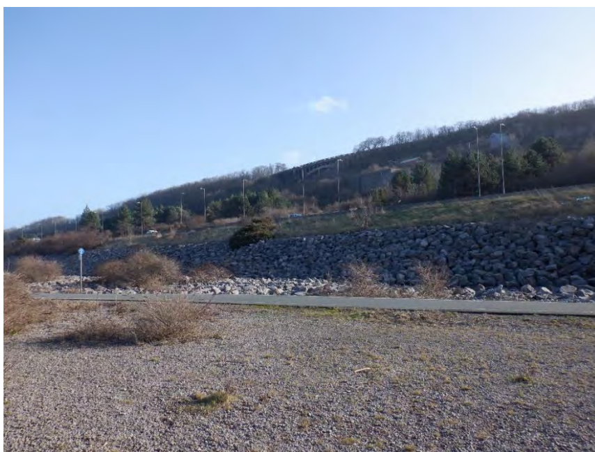
Plate 4 – View to the south of the foreshore in CMU 3-1 looking at the A55 and its rock revetment facing south east.
