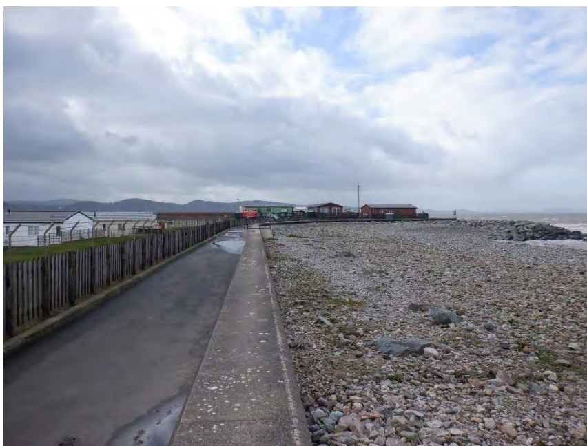
Plate 35 – The view looking west across CMU 3-5B
