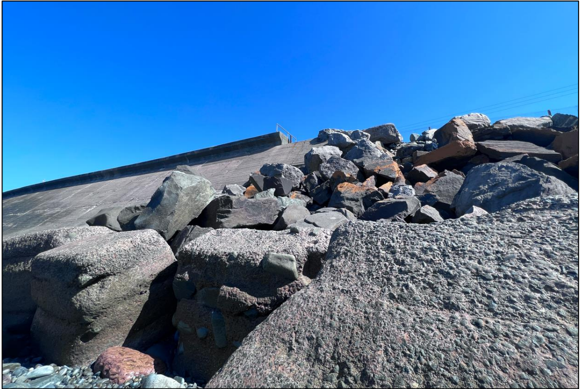
Figure 6: Rock armour interfaces with end of formalised hard defence wall.
