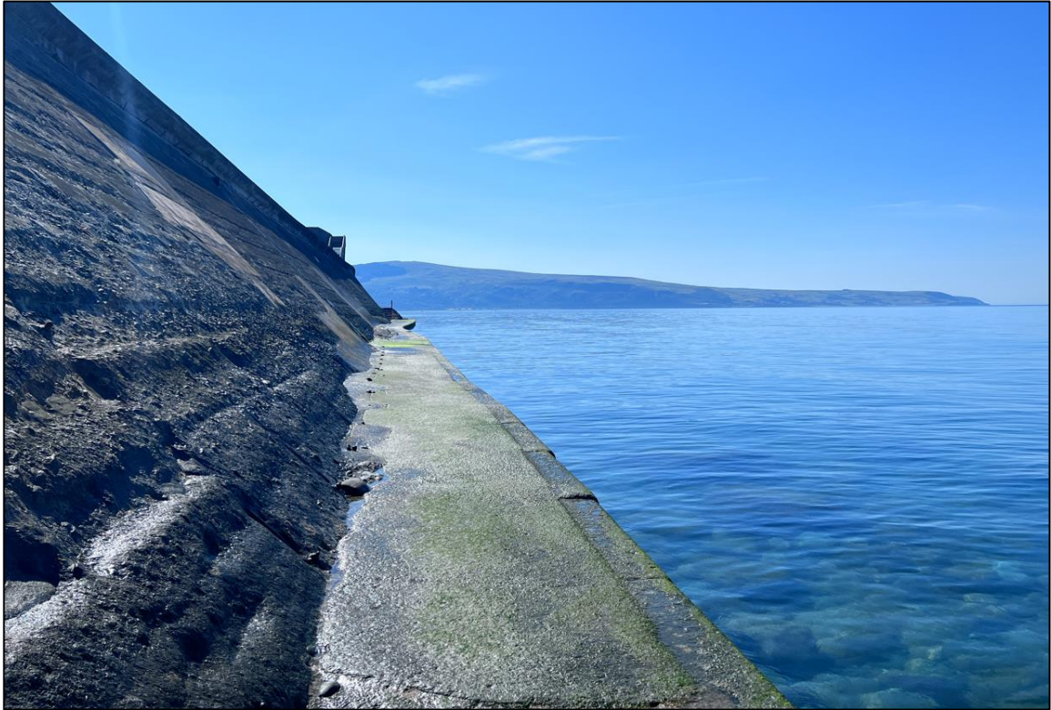
Figure 4: View of lower defence toe reinforcement below Llanaber Station.
