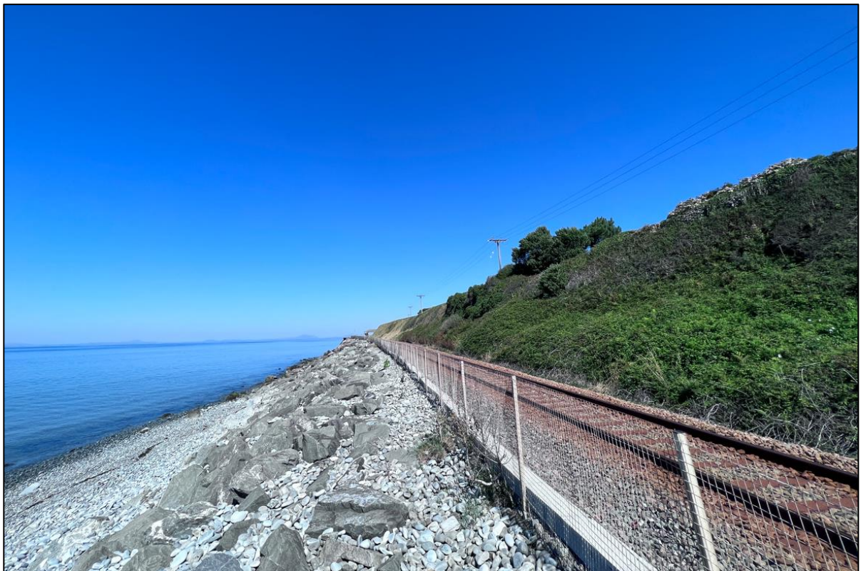
Figure 9: Vegetated embankment behind armour and pebble beach.
