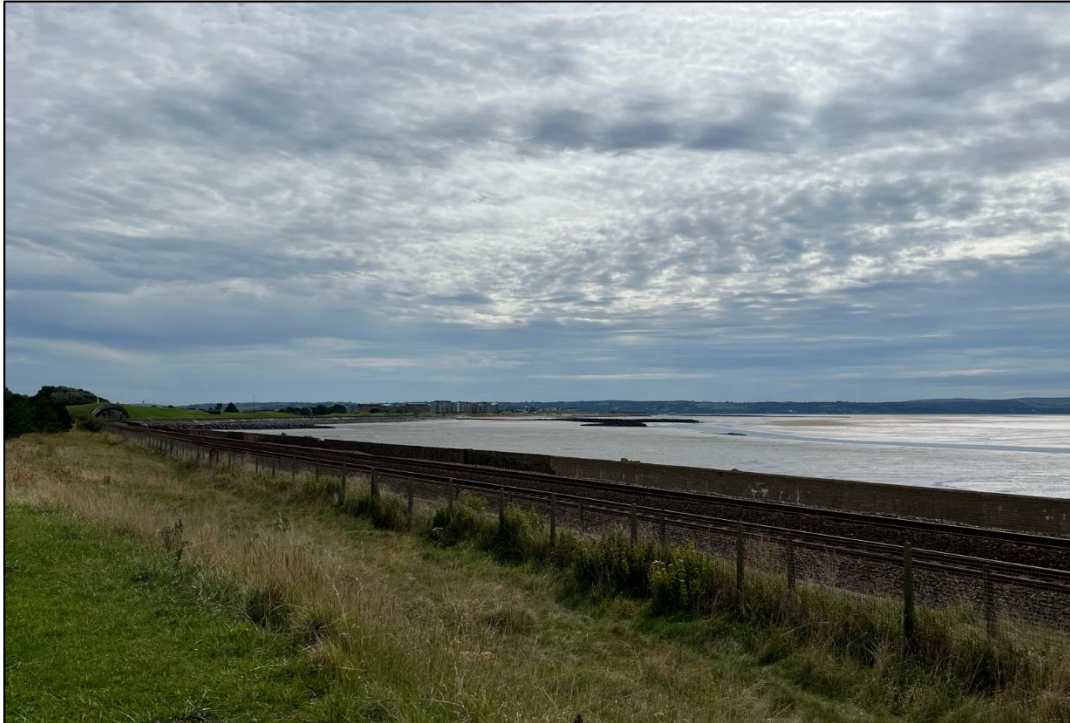
Figure 4: Rear of sea wall behind network rail boundary.
