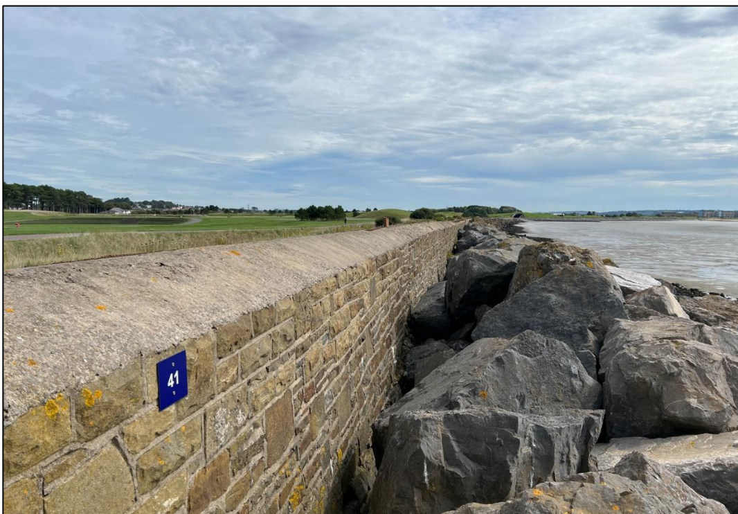
Figure 5: Seawall defence protected by significant rock armour embankment.
