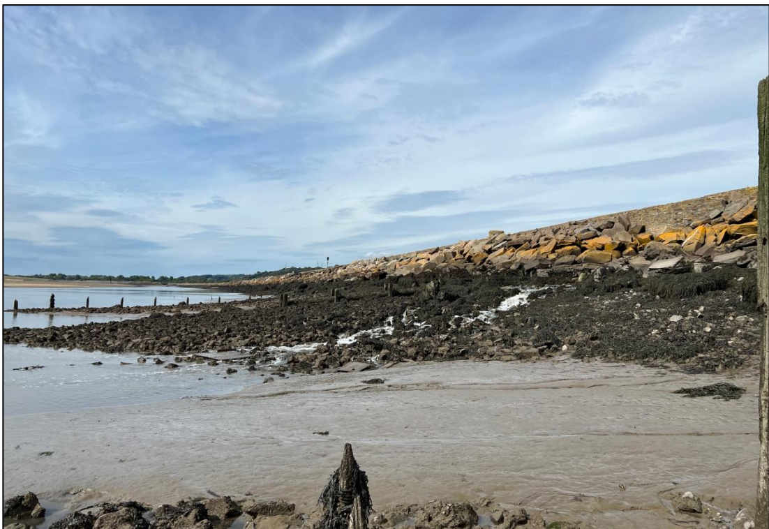
Figure 7: Outfall situated between rock armour and defence wall.
