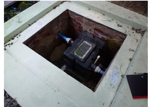
Water flows under gravity through the collection / inspection chambers and into the tanks then water is pumped to the factory if it is to be used in process. If water is not to be used in process it is discharged under gravity from the plastic collection tank.
