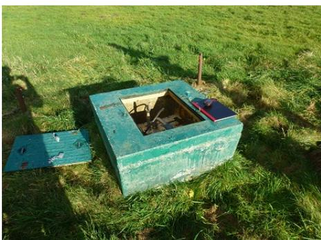
The borehole headworks are located in a brick lined, above ground chamber with a manhole cover. The borehole headworks is manufactured from stainless steel and is loosely bolted to a mild steel casing/upstand, (diameter could not be measured). The borehole is understood to be approximately
