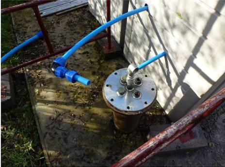
The borehole comprises a plain plastic casing to a depth of approximately 6mbgl beneath which the borehole comprises slotted plastic well screen to a depth of approximately 38mbgl. The bottom ~1m of the borehole comprises plain plastic casing. The borehole headworks is completed above ground, with a mild steel upstand and stainless steel well plate.
