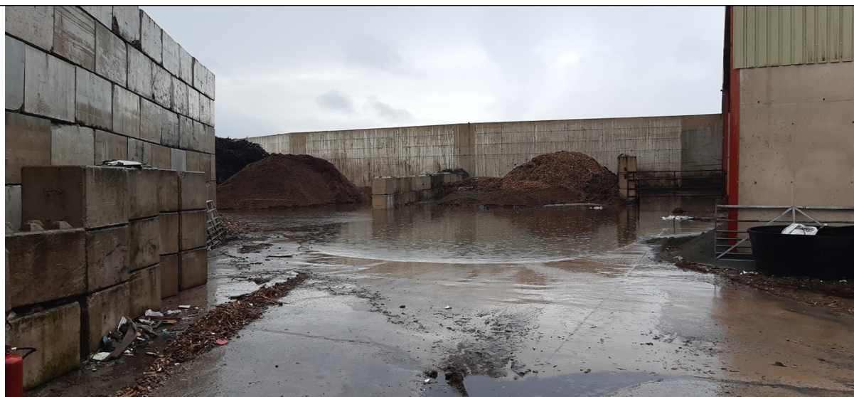
Photo 6 - Photo of fire incident taken by NRW Officer Greg GARDNER on 01/11/22
