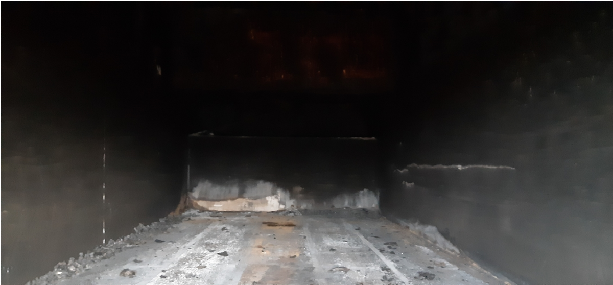
Photo 4 - Photo of fire incident taken by NRW Officer Greg GARDNER on 01/11/22
