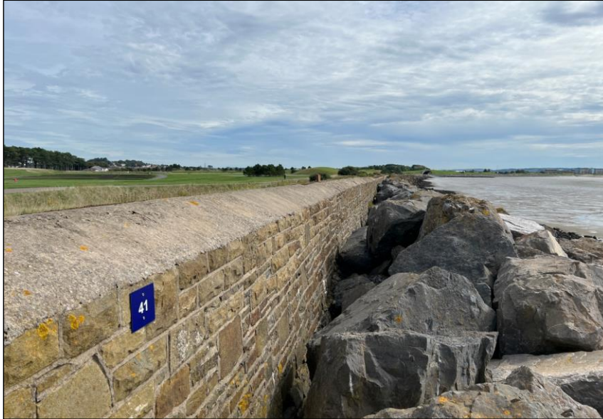
Figure 7: Seawall defence protected by significant rock armour embankment.
