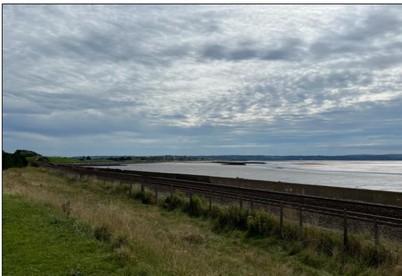
Figure 6: Rear of sea wall behind network rail boundary.
