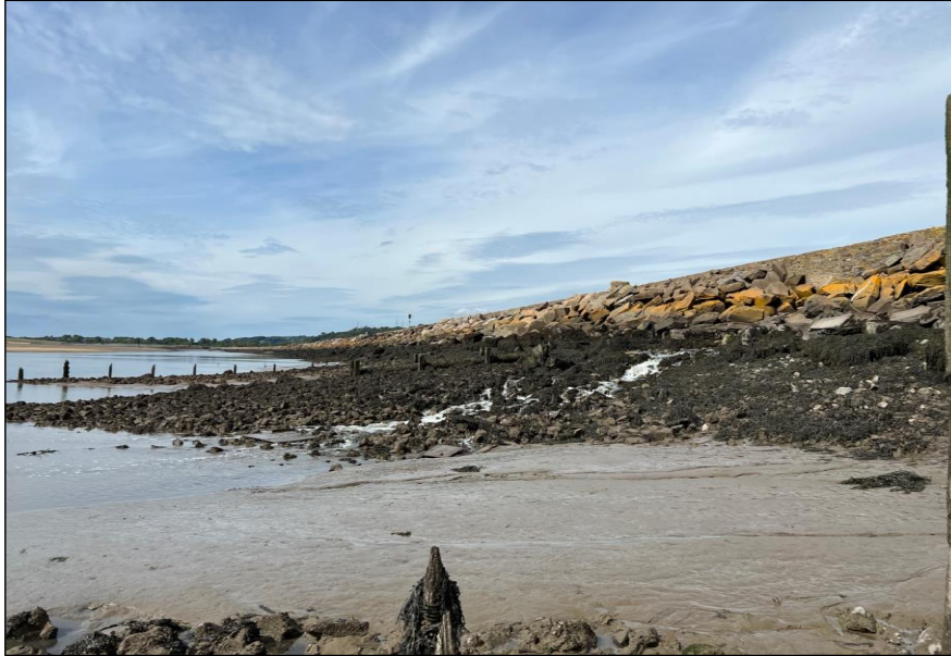
Figure 9: Outfall situated between rock armour and defence wall.
