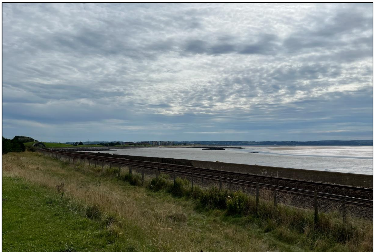
Figure 5: Rear of sea wall behind network rail boundary.
