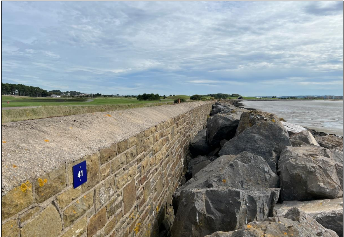
Figure 6: Seawall defence protected by significant rock armour embankment.
