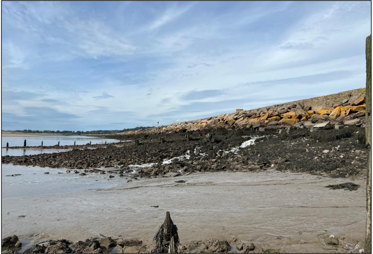
Figure 8: Outfall situated between rock armour and defence wall.
