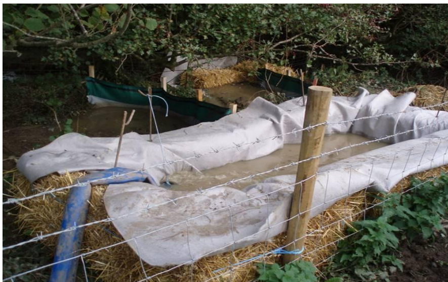
Figure 9: Bale and Geotextile Sump
