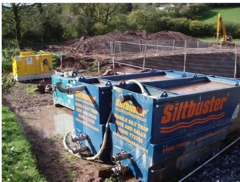
Figure 10: Pumping silt contaminated water through Lamella Clarifiers
