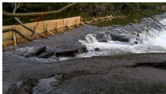
Plate 8-27. Poor condition of the weir including the baulk fish pass, looking from the RHB concrete apron
