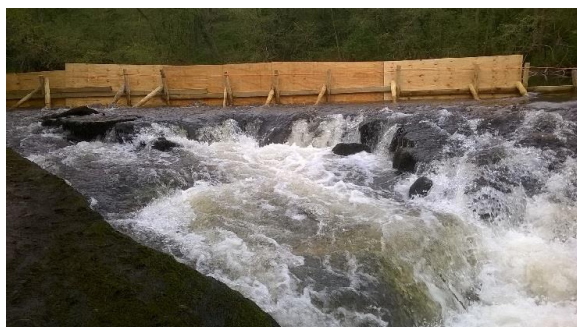
Plate 8-26. Poor condition of the weir, looking from the RHB concrete apron
