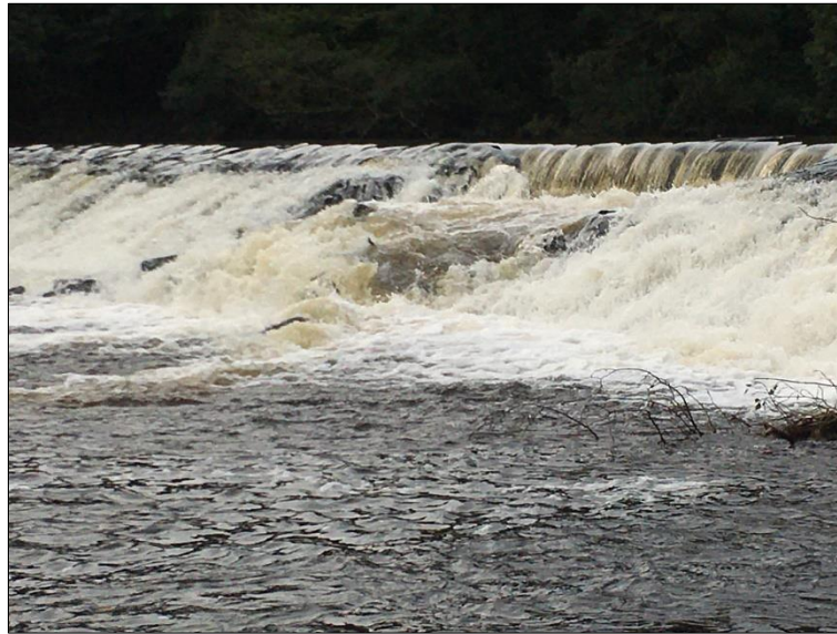
Figure 9: Collapsed section in the centre of the weir
