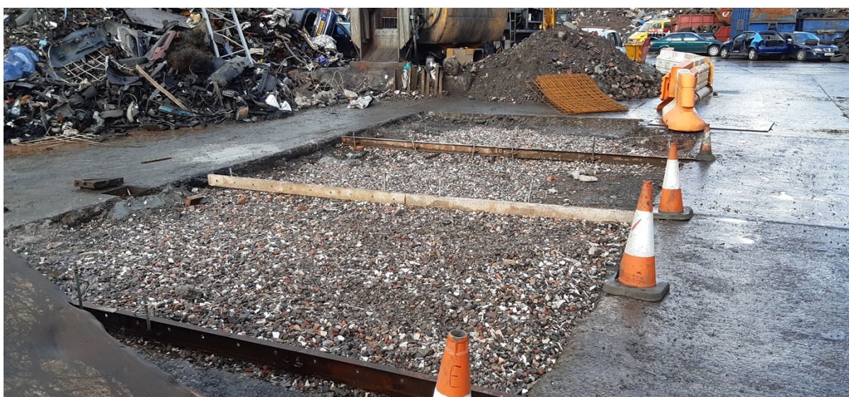
Photo 2 - Flooring infrastructure improvements at Fred Lloyd & Sons
