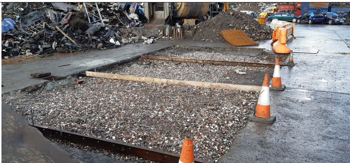
Photo 2 - Flooring infrastructure improvements at Fred Lloyd & Sons
