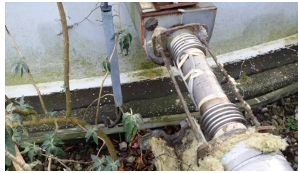
Intrusion into pipework casing
