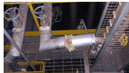
Intrusion into pipework insulation
