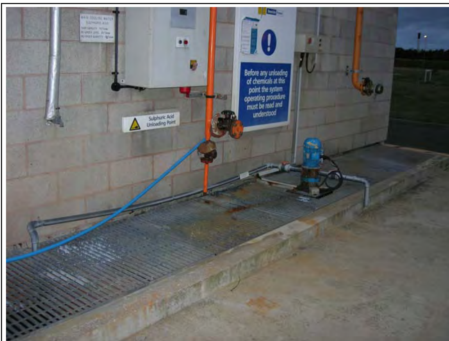
Photo 6: Contained sulphuric acid unloading area.
