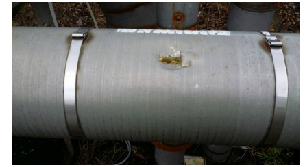
Intrusion into pipework casing
