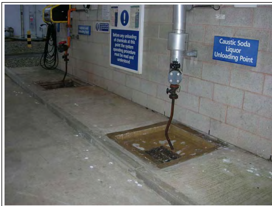
Photo 3: External fill point for sulphuric acid and caustic soda, sited on external wall of water treatment plant.
