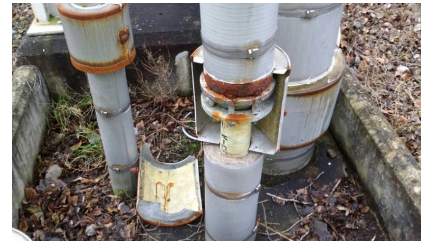
Inspection of pipework flange
