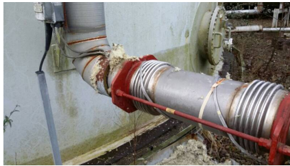
Intrusion into pipework casing
