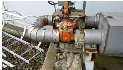
Inspection of pipework flange
