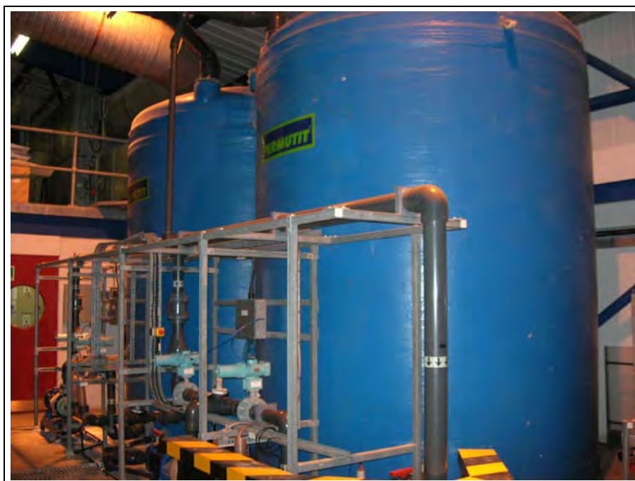
Photo 4: Internal sulphuric acid and sodium hydroxide storage tanks within the water treatment plant
