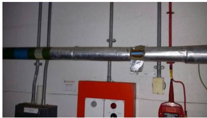
Intrusion into pipework insulation
