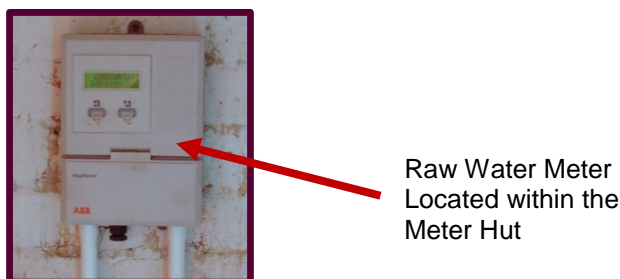
Figure 2. Raw Water Meter
