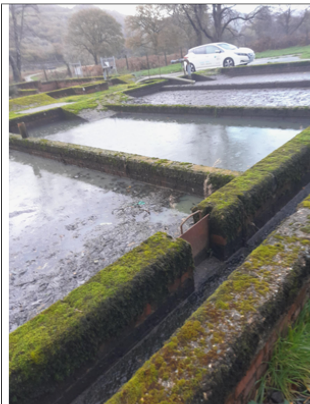
Image of the 3 sludge tanks.
