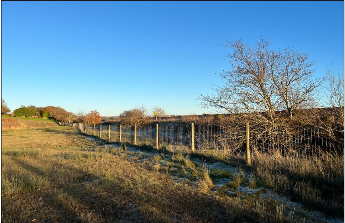
Figure 8: North Side, 100m south of Culvert.
