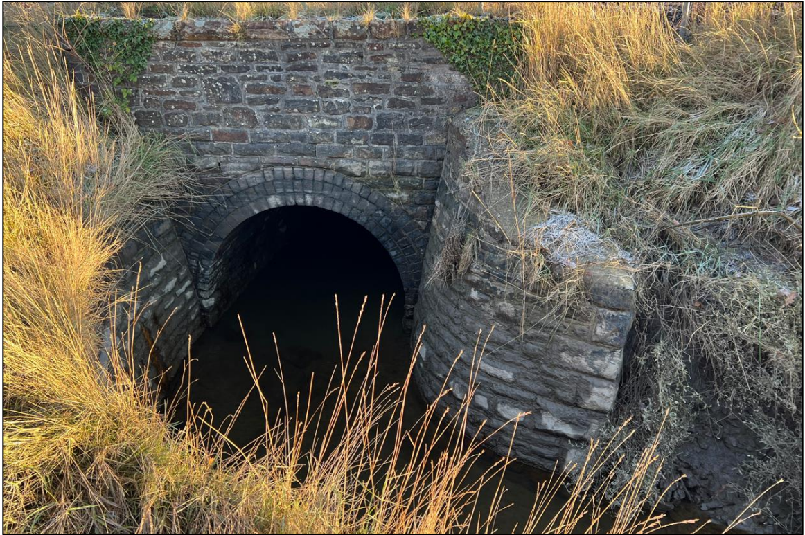
Figure 6: Inlet of culvert below rail corridor (north side).
