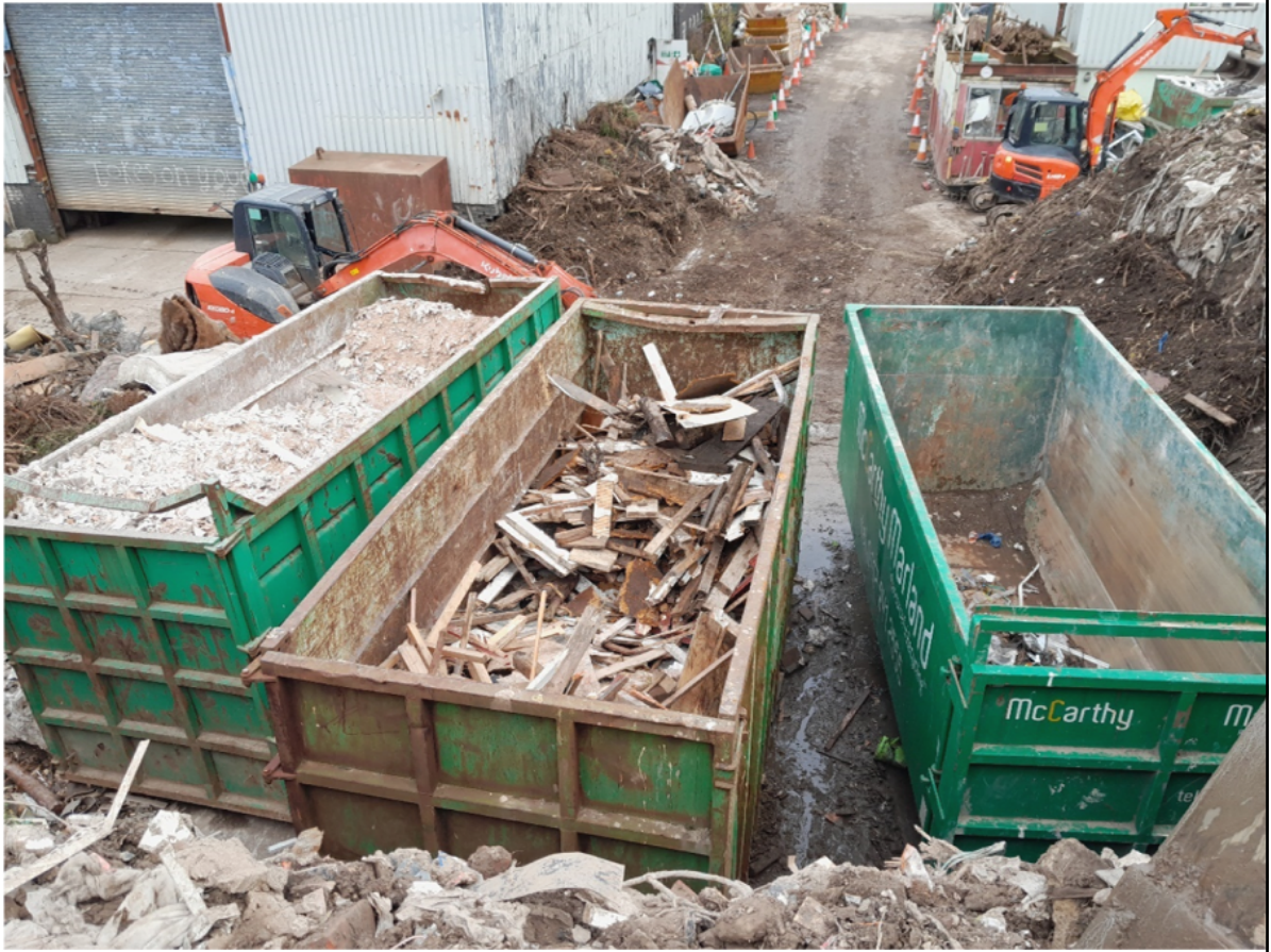
Image showing the skips, containing plasterboard, wood & general waste (Image 4)
