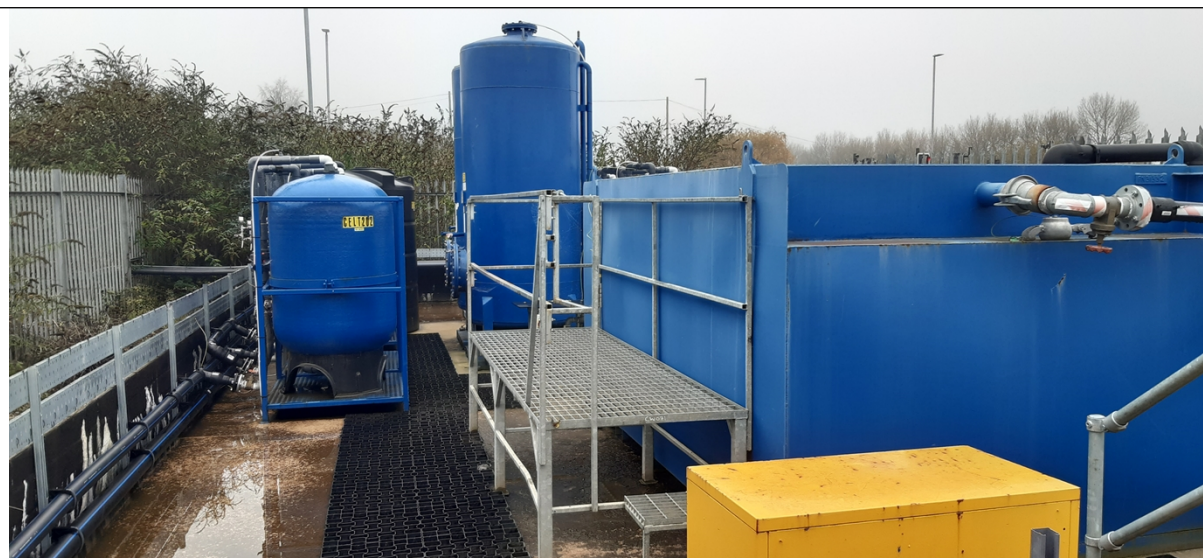
Photo 2 - Concrete bunded wall (bottom left foreground in black)
