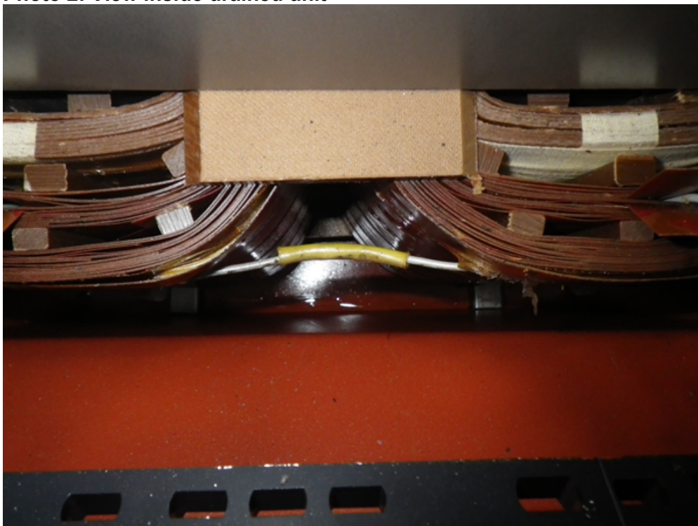
Photo 2: View inside drained unit
