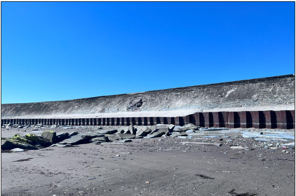
Figure 9: Additional sheet pile protected defence toe.
