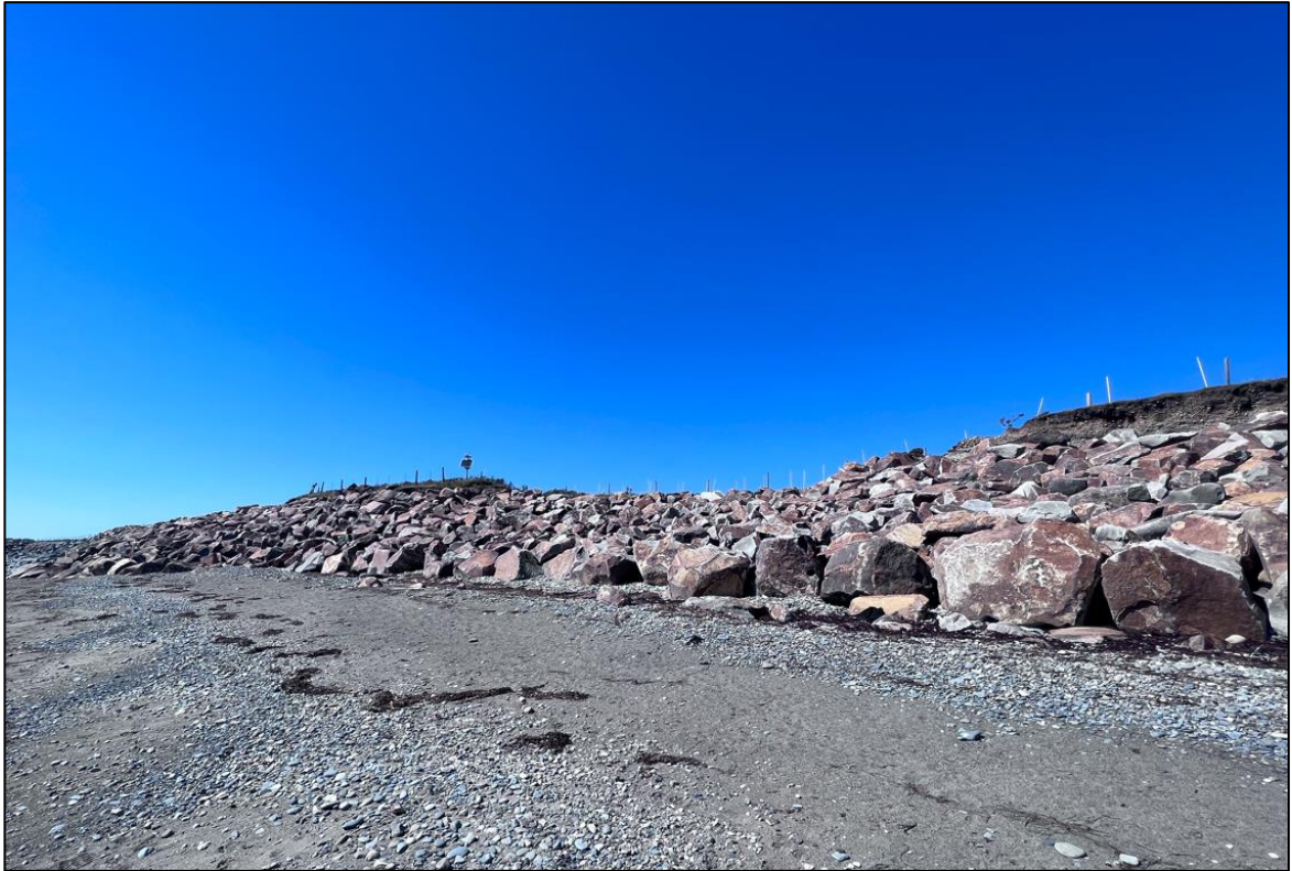
Figure 6: New rock armour towards the most easterly section of the defence.
