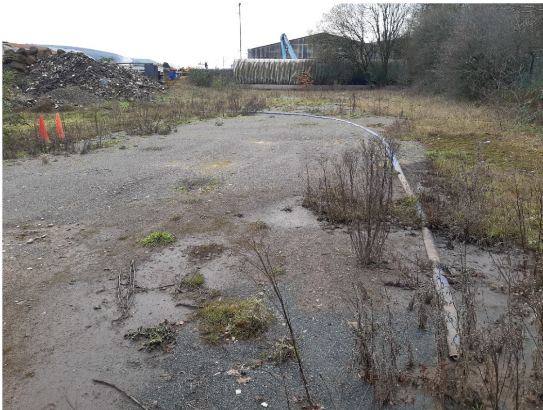
Photo 2 – hose leading from drainage channels within the operational storage area of the yard.
