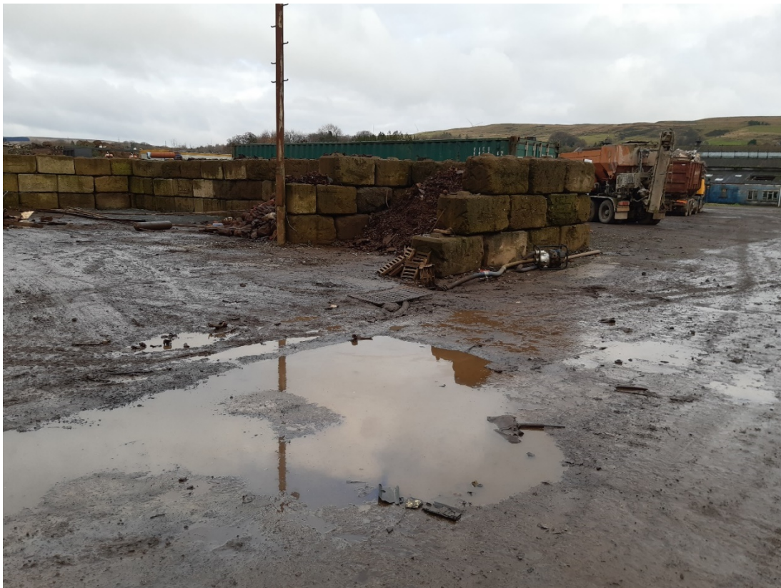
Photo 1 – Storage area with standing surface water with pump in-situ.
