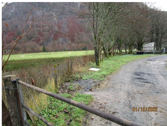
Photo showing STW's perimeter fencing
