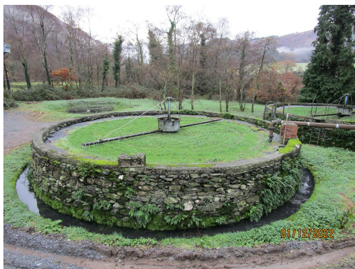
Photo of grass growth on surface of filter beds.
