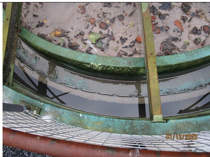
Photo showing organic matter growth in primary tank.
