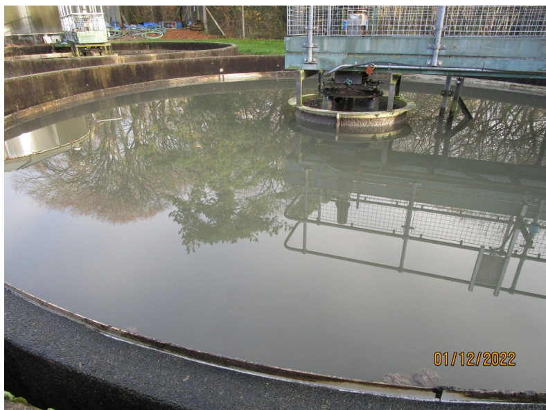
Photo 1 - Criccieth storm tanks during OSM inspection
