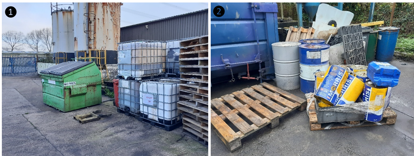
Photograph 1 & 2: IBCs and drums storing waste oil/lubricant not provided with secondary containment.
