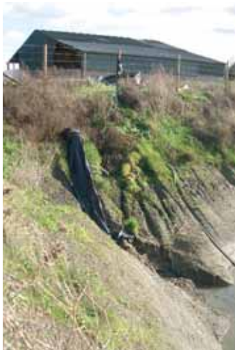
Some erosion problems have been experienced as the rainwater drains in to the lagoon
