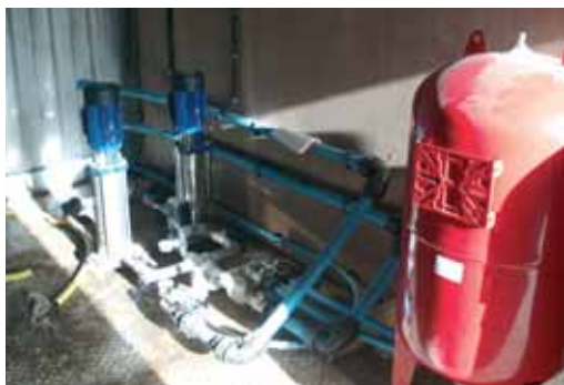
Pumps and pressure vessels in the Oakey Farm 'pump room container body'
