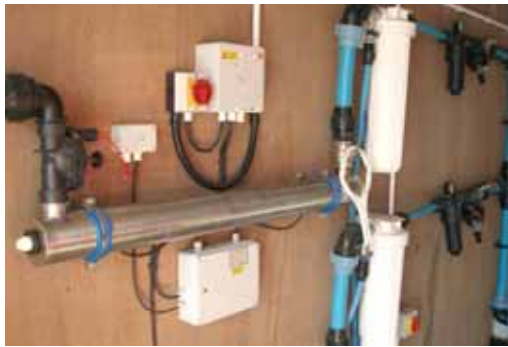
Water filters and UV water treatment at Oakey Farm
