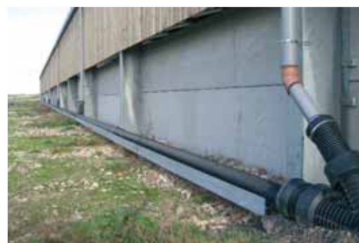
The down pipes collecting rainfall off the cubicle building – no filtration at this stage as the water is drained direct to a lagoon
