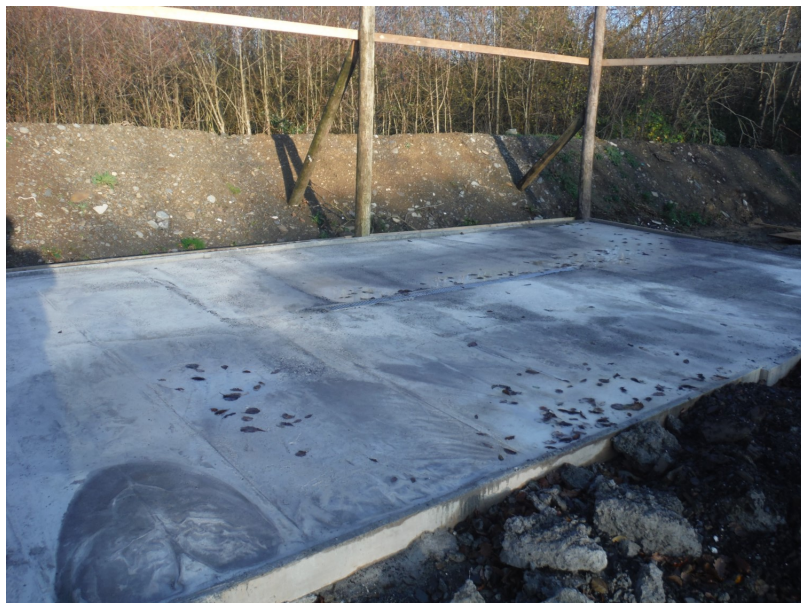
Photo 2 - Concreted ELV Depollution Bay
