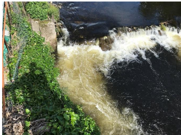
Plate 5-11. Weir from RHB (turbulent flows apparent at RHB end/ weir broken up at this location)
