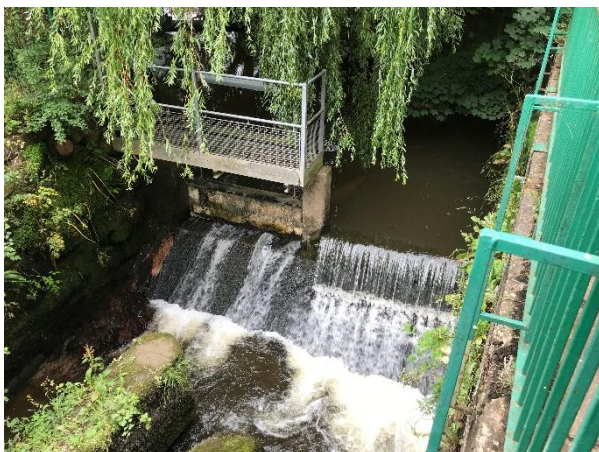
Plate 8-6. Flow structures at top of the leat channel (penstock lowered)
