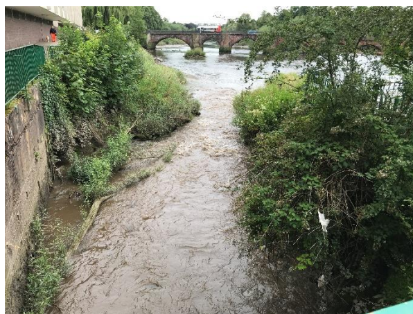
Plate 8-9. Leat channel looking downstream (penstock raised allowing more flow down it)
