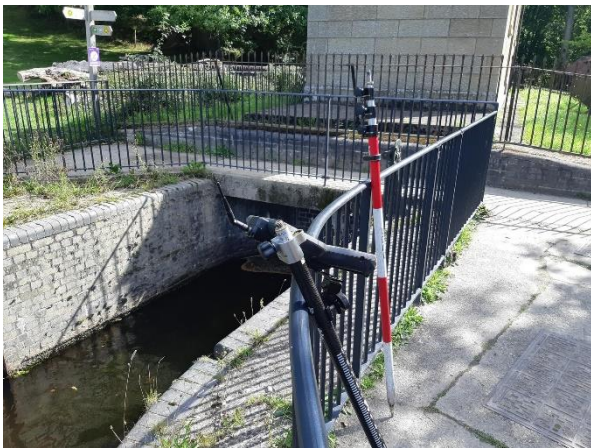
Plate 3-9. Building above the channel feeder stream, under which channel is culverted and flow is monitored
