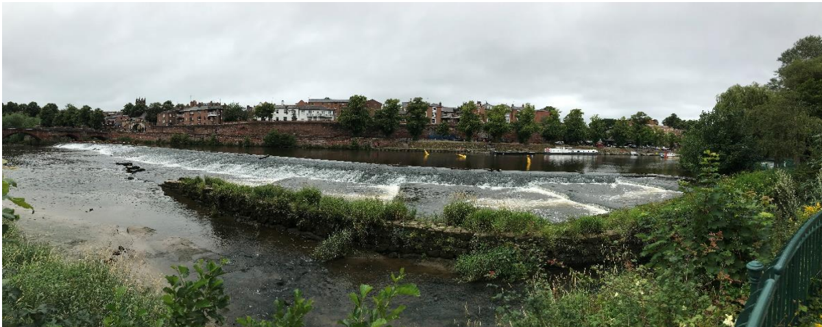
Plate 8-1. View across channel/ weir/ fish pass (from RHB)- dilapidated fish pass walls evident at downstream end
