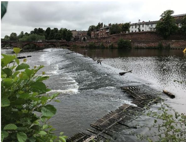
Plate 8-2. Top of fish pass (oversails apparent)
