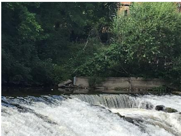
Plate 7-6. Broken up section toward the LHB side of the weir
