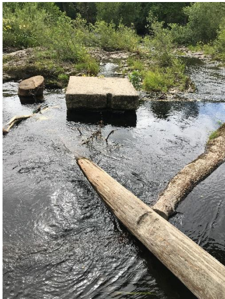
Plate 3-2. Structure in channel at weir (one end of where stoplogs can be inserted to dry up channel to canal for when that is maintained)
