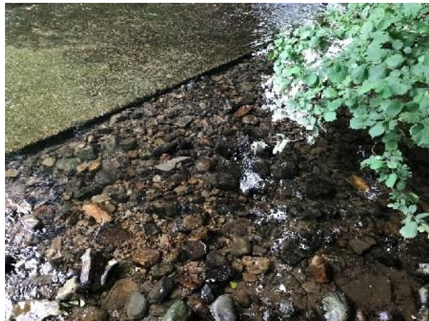
Plate 6-6. Upstream of the ford, showing sediment, gravels and stone build up
