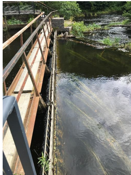
Plate 3-3. Screens at entrance to canal feeder stream
