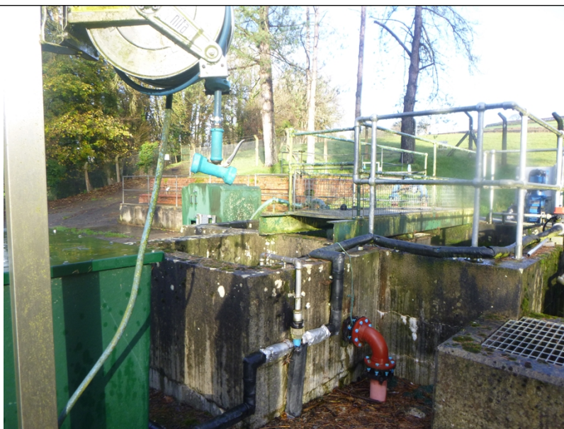
Photograph 2: Primary Settlement Tank (PST)
