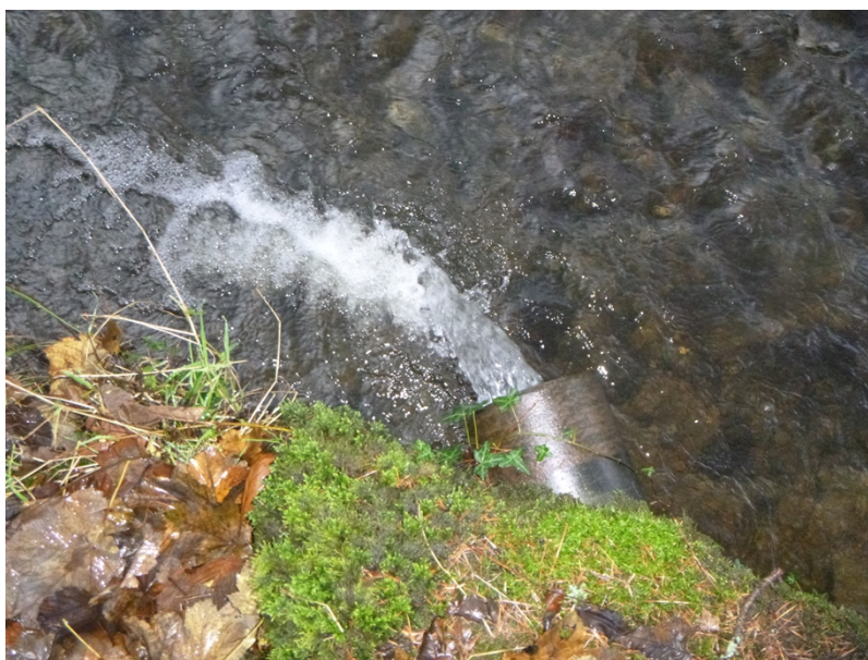
Photograph 9: Final effluent outfall into the Afon Grannell
