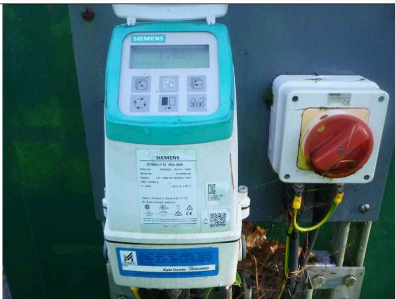
Photograph 8: MCERTS flow measurement system
