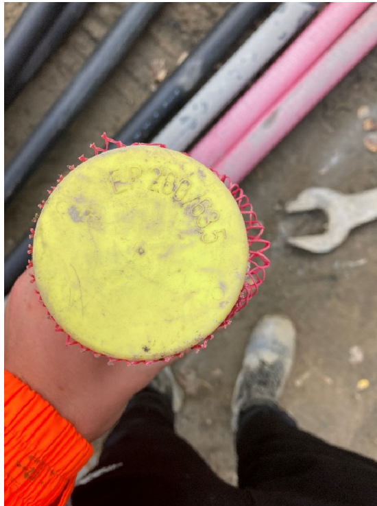
Photograph 3 Push-fit end cap supplied for the works
