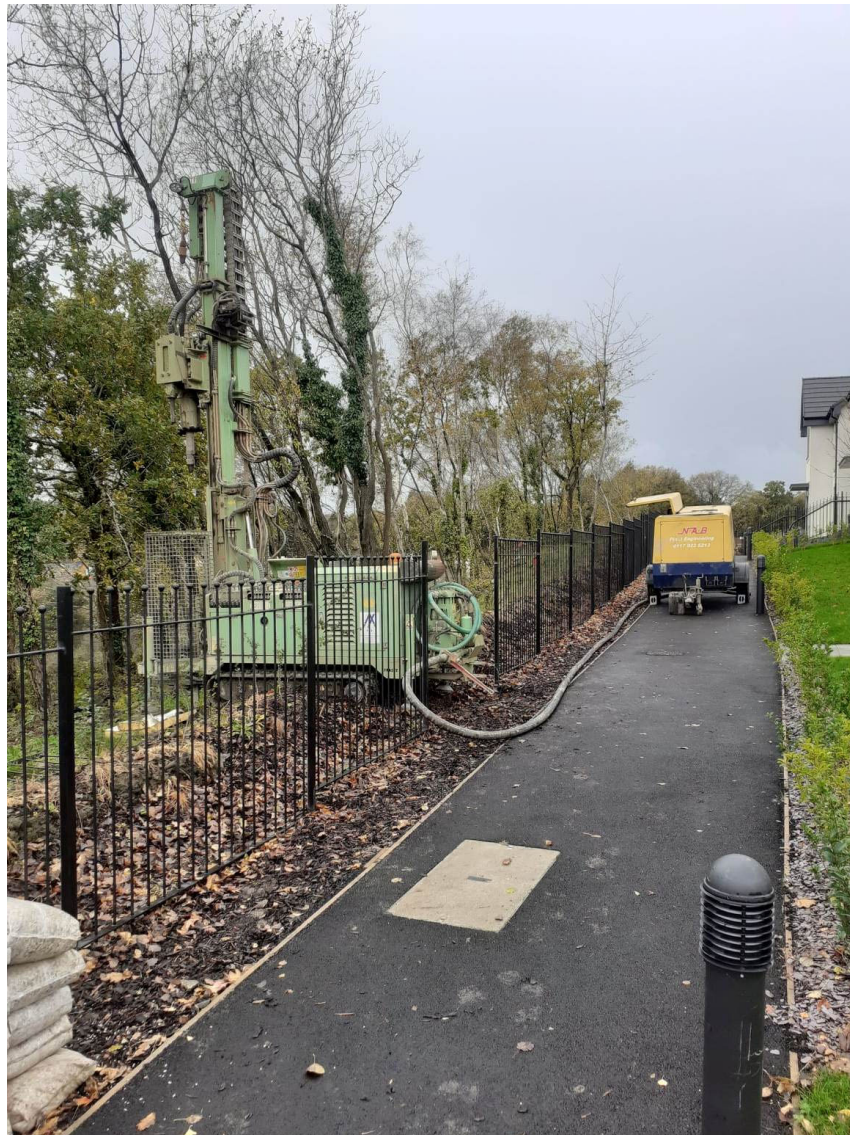
Photograph 8 Rotary open hole drilling rig on position at borehole LFG23R
