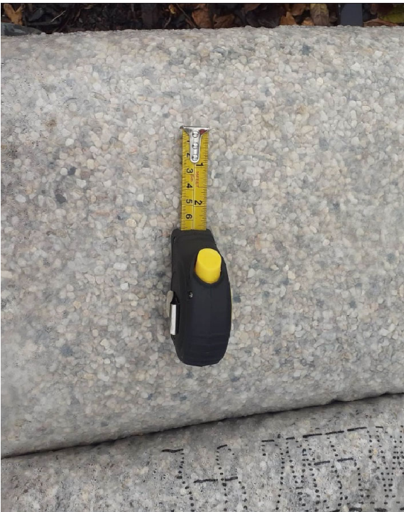
Photograph 1 3-6mm filter gravel supplied for the works
