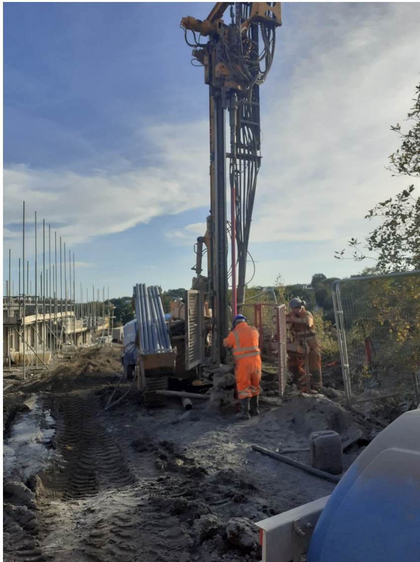
Photograph 7 Rotary open hole drilling rig on position at borehole LFG44R
