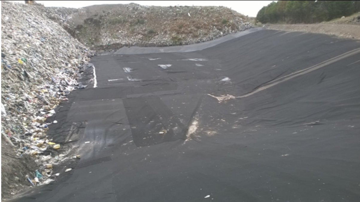
Photo 6 showing sub cell construction
