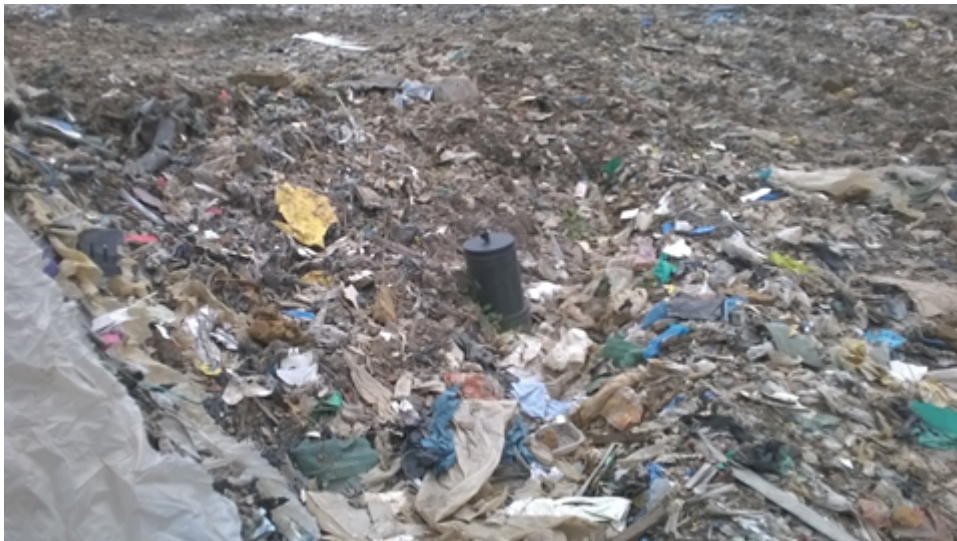
Photo 5 showing In-waste lfg / leachate well 2
