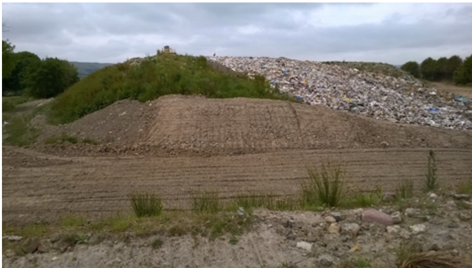
Photo 1 showing sub cell 5 tipping.
