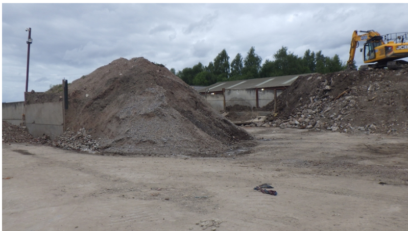
Inert stockpile height against concrete walls.
