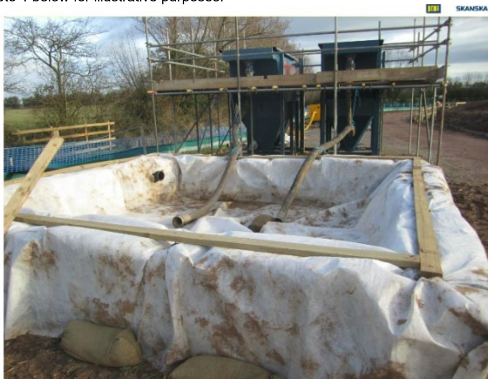
Photo 1 – Typical Silt Trap constructed of straw bales and geotextile membrane.
