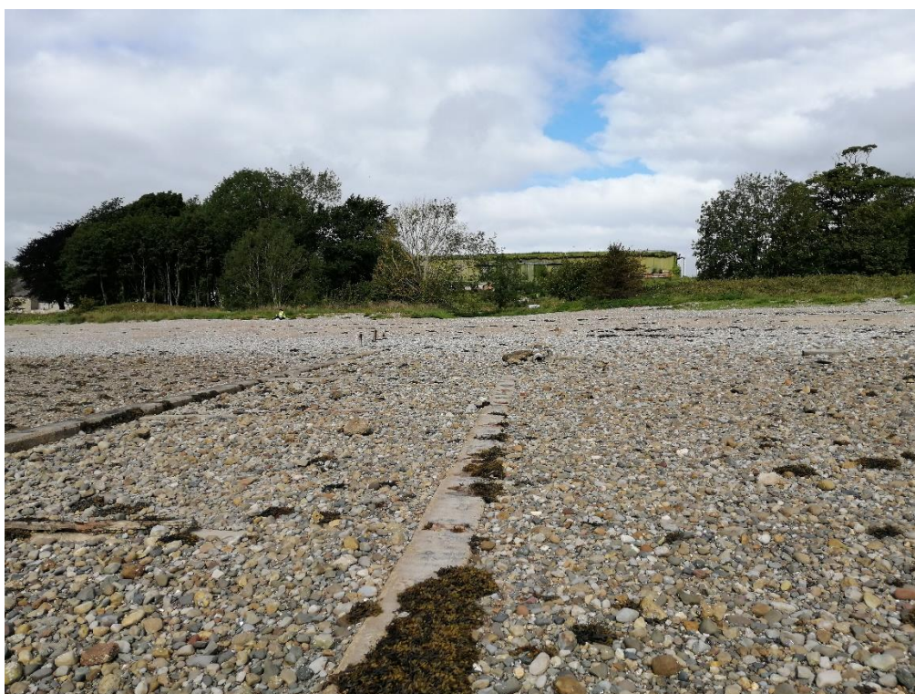
Photograph 1 Looking landward towards outfalls 1 and 2.
