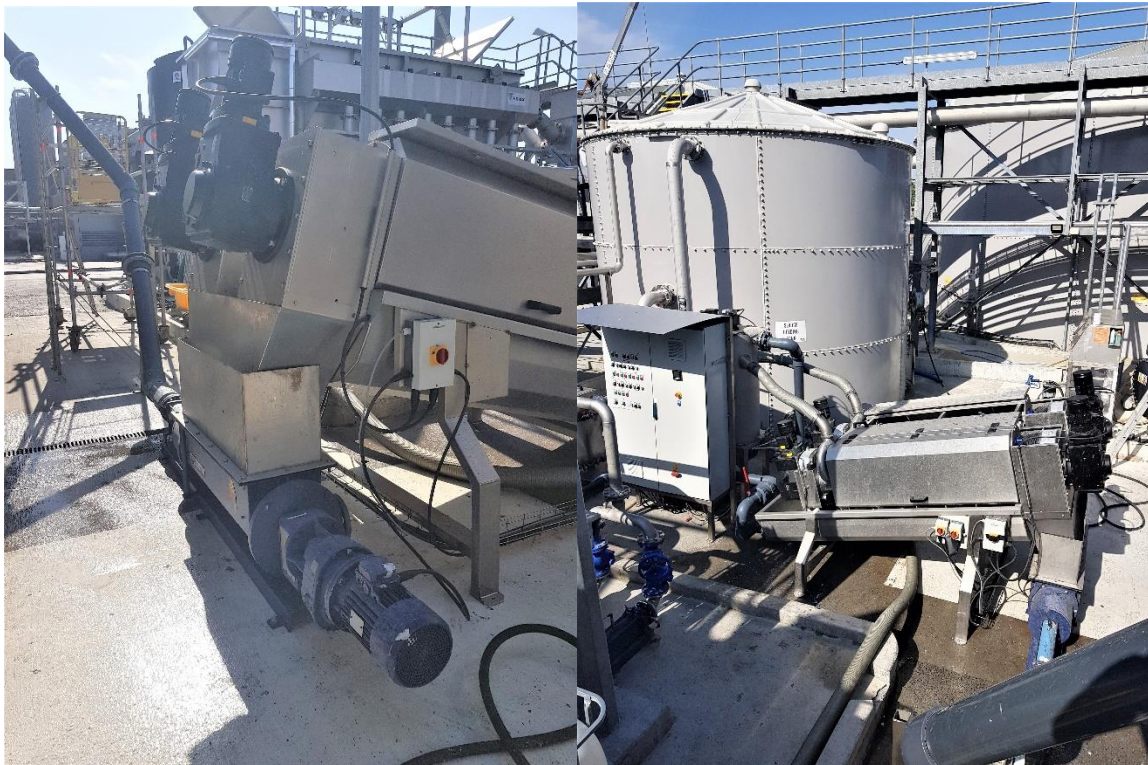
Glanbia Belview Hydro Double 400 Screw Press mounted at low level discharging into a Sludge Cake Pump
