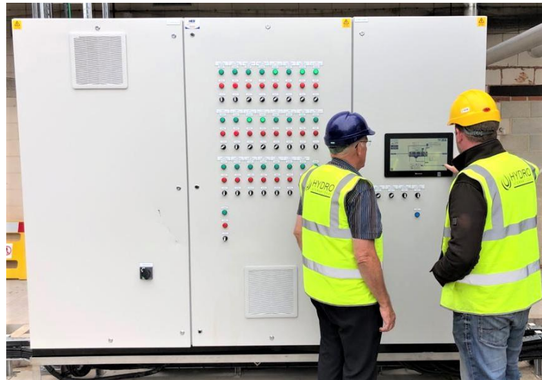
Control Panel with PLC & HMI Creative Foods Burton-on-Trent, UK
