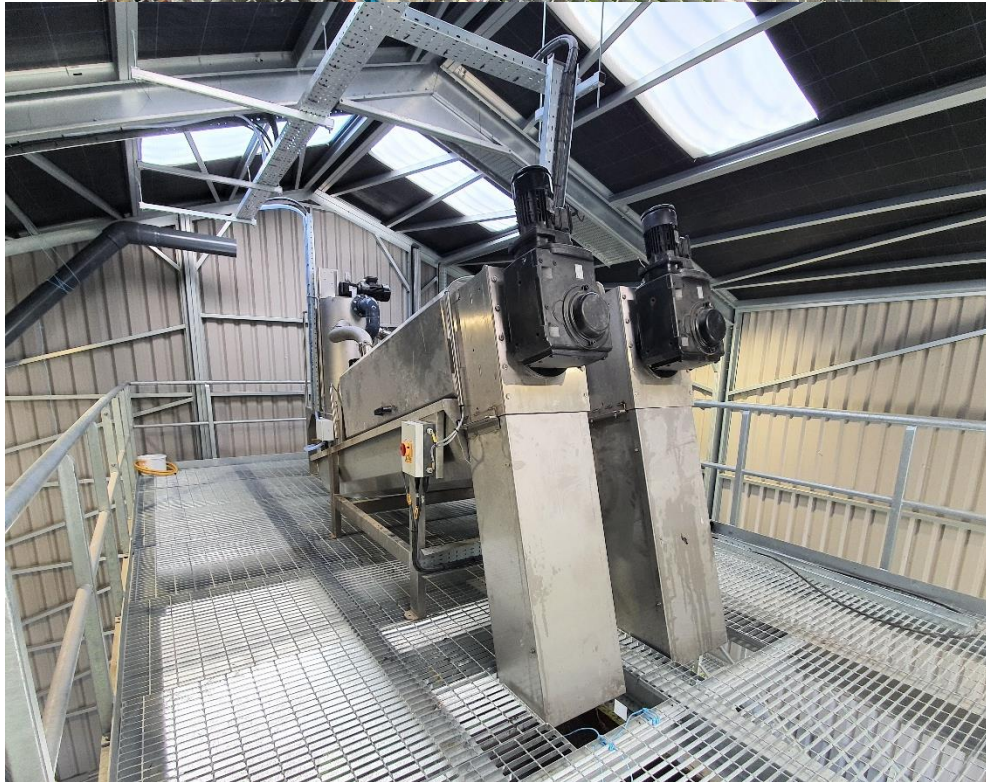
Double Hydro 400 Screw Press on high level platform inside a Building
