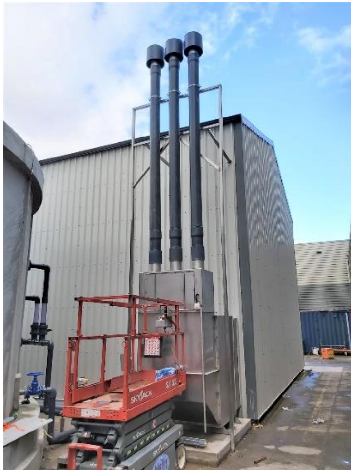
Odour Carbon Filter recently installed on the Sludge Dewatering Building, Keurig Dr Pepper WWTP, Newbridge, Co. Kildare
