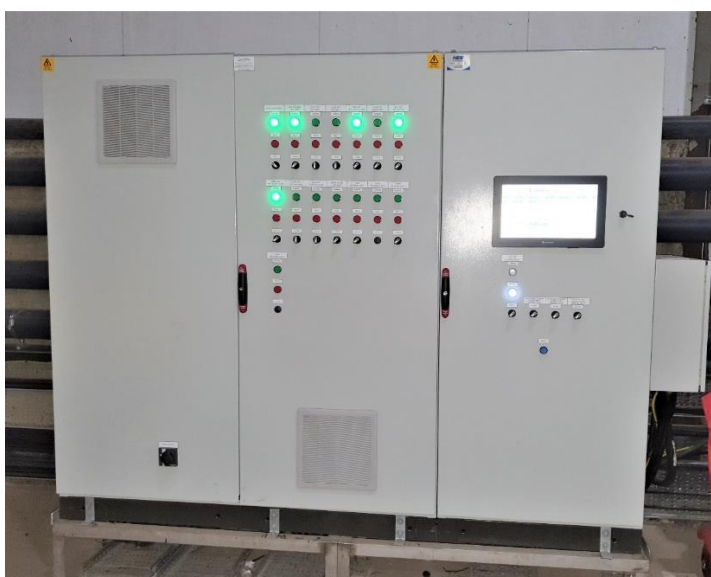
Control Panel with PLC & HMI Plastics Recycling facility Cotesbach, Rugby, UK
