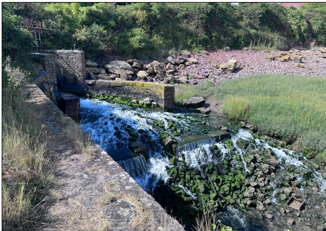
Figure 5: Tidal flap protection walls and outfall stream.
