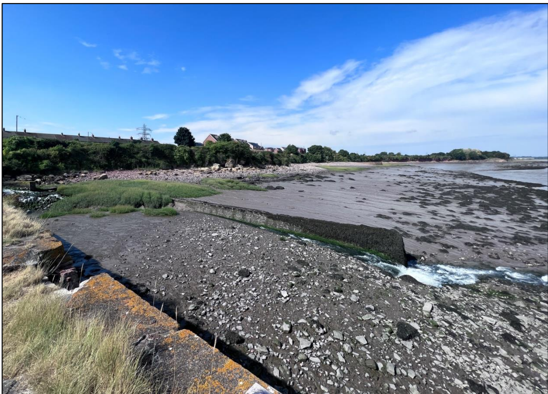
Figure 7: Smaller dwarf defence wall aiding channel of Sudbrook outfall water.
