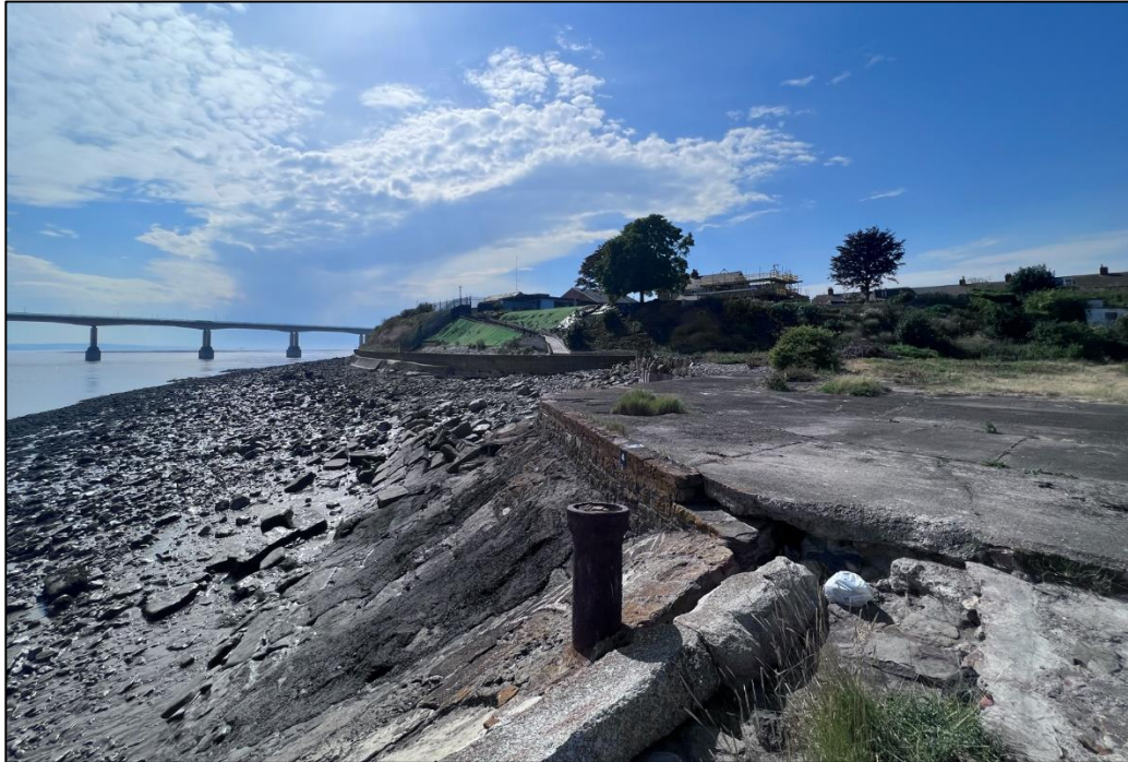
Figure 4: Upper section of sea defence upstream of slipway onto beach.
