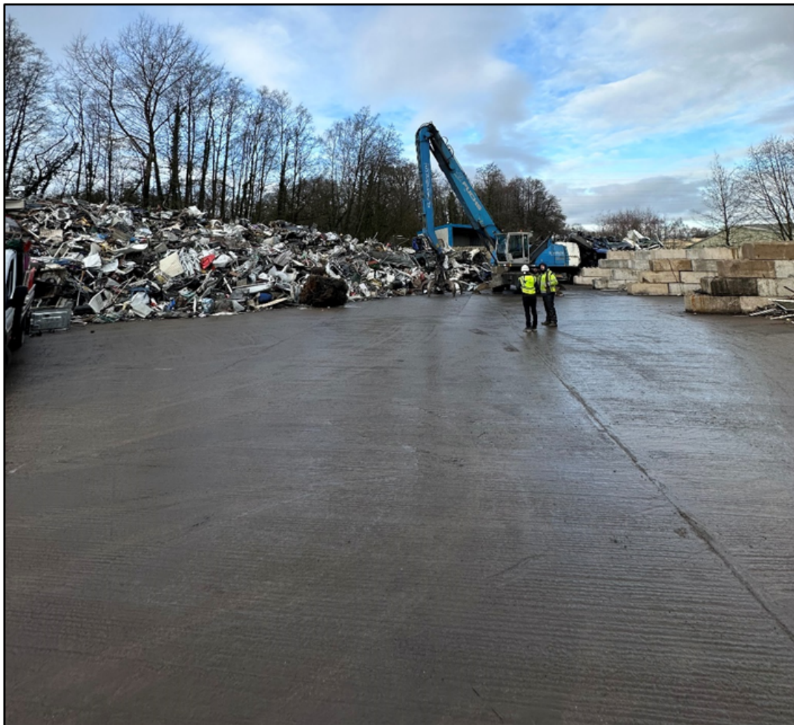
Image 1 - showing the re-surfaced yard with compliant waste volumes on site
