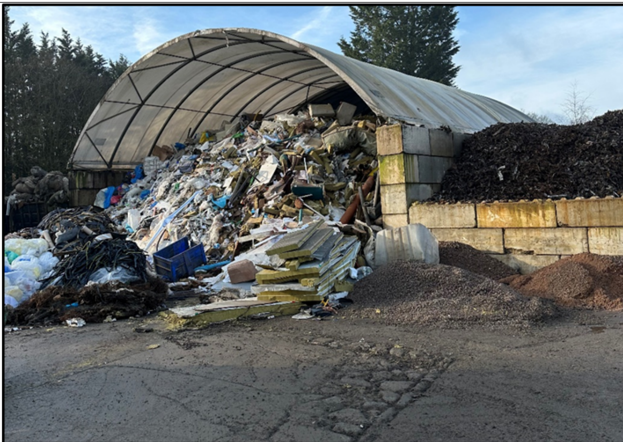
Image 4 - showing transfer station zap shelter filled with mixed municipal waste
