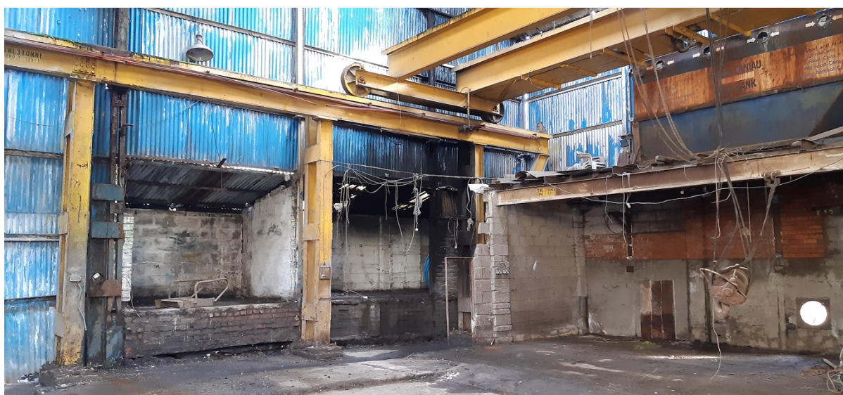
Photo 1 - Site cleared at ADJ Skip Hire Ltd
