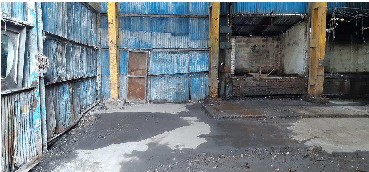
Photo 3 - Site cleared at ADJ Skip Hire Ltd
