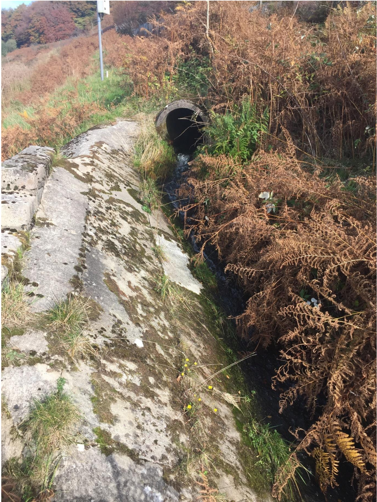
Existing structure at intake location showing underground pipe surfacing
