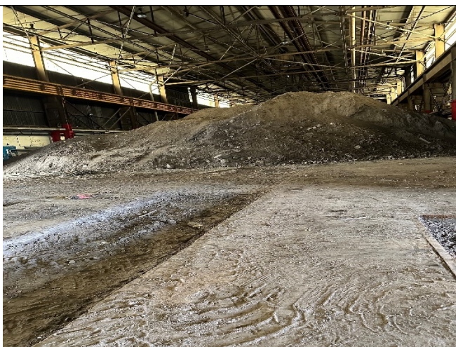
Image 3 - showing waste material stored within the building
