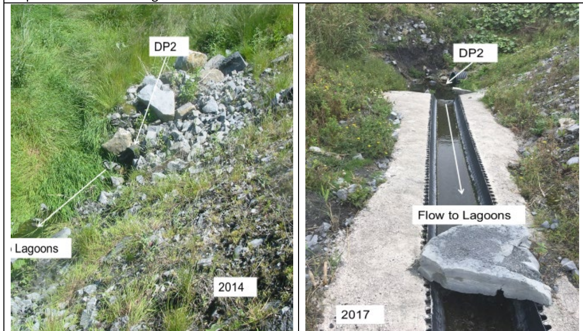
Improvements to DP2
