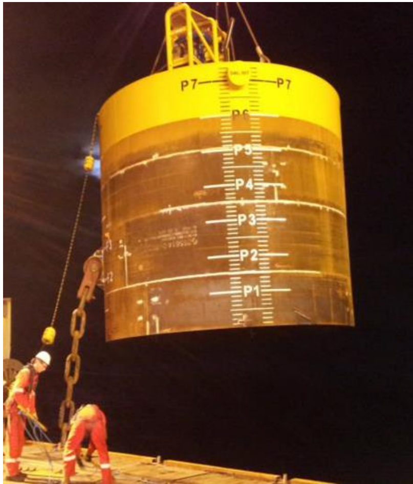
Figure 4.1: Suction bucket foundation
