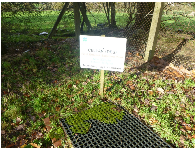
Photograph 5: Final effluent sampling point
