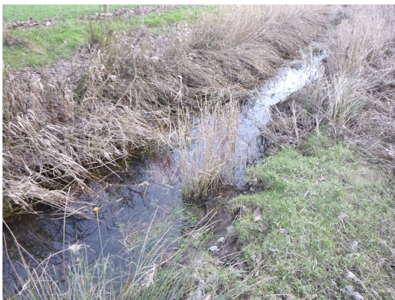
Photograph 7: Drain to the Afon Teifi
