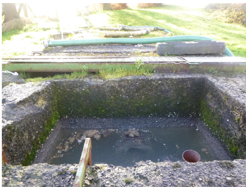
Photograph 1: Septic tank (background) and chamber (foreground)
