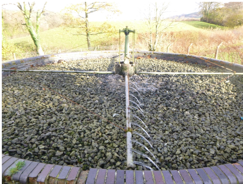
Photograph 3: Stone media filter bed (post arm clearing)
