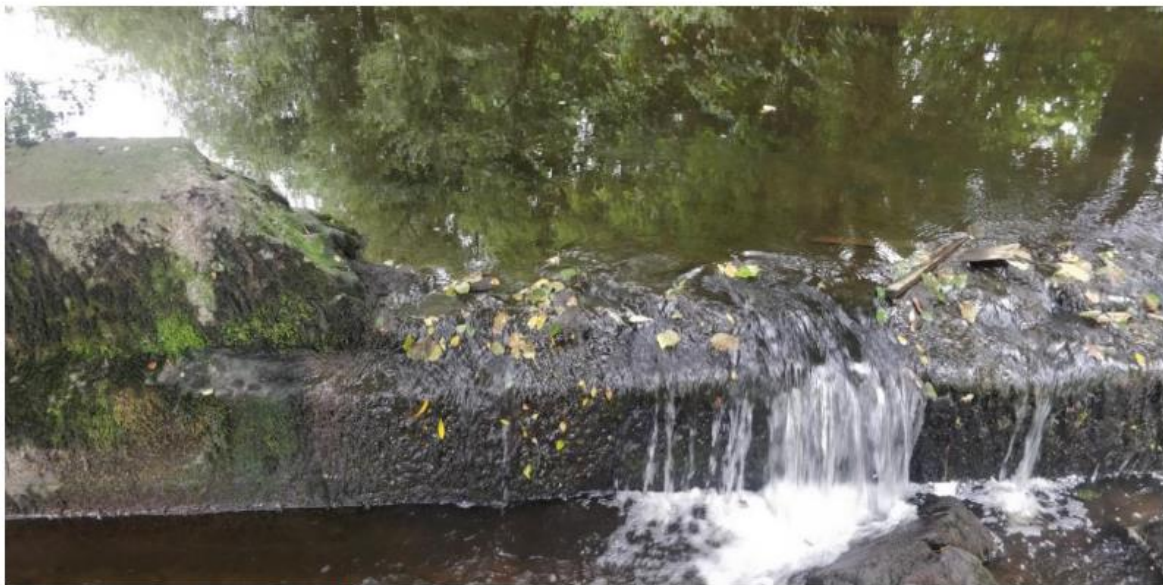
Figure 3. The weir is constructed from concrete.
